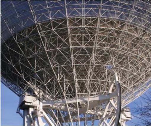
**Fig. 9.29.a** Effelsberg 100-m telescope. The picture shows the rear side of the OPEN BUS fully exposed to the thermal environment [Courtesy N. Junkes, MPIfR, Germany].
