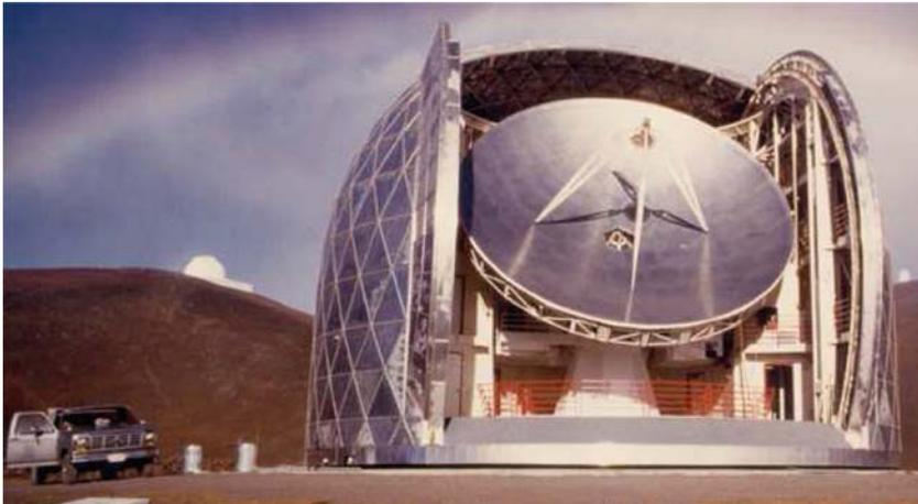
**Fig. 3.2** Astrodome of the 10-m Caltech Submillimeter Observatory Telescope (CSO, Hawaii, 4 000 m altitude). The astro-dome is opened at night for observations [Image courtesy Sub-mm Observatory, USA. Picture taken by R. Howard, CSO Site Manager].
