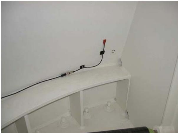
**Fig. 6.1** PT 100<sup>TM</sup> electric resistance temperature sensor installed inside the VertexRSI ALMA 12-m prototype antenna. Although the sensor is located at one spot, due to good thermal conduction of the metal wall the measured temperature is representative for a large area [Courtesy N. Emerson, NRAO, USA].
