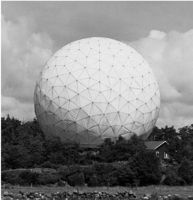
**Fig. 3.4** Radome of the 20-m Onsala Space Observatory Telescope (OSO, Sweden, sea level). The radome consists of Goretex<sup>TM</sup> plastic material supported by a space frame and overpressured inside air [Courtesy L.E.B. Johansson, Onsala Observatory, Sweden].
