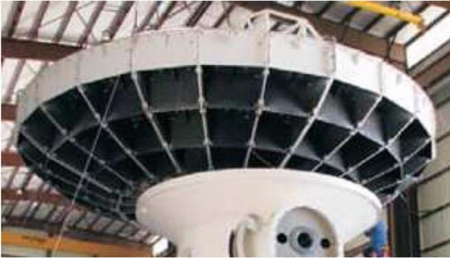
**Fig. 9.29.c** ALMA VertexRSI 12-m telescope. Illustration of a CLOSED BUS (the rear cladding is taken off) built from plates forming COMPARTMENTS. Natural convection inside the compartments is small [Image Courtesy of NRAO/AUI/NSF].
