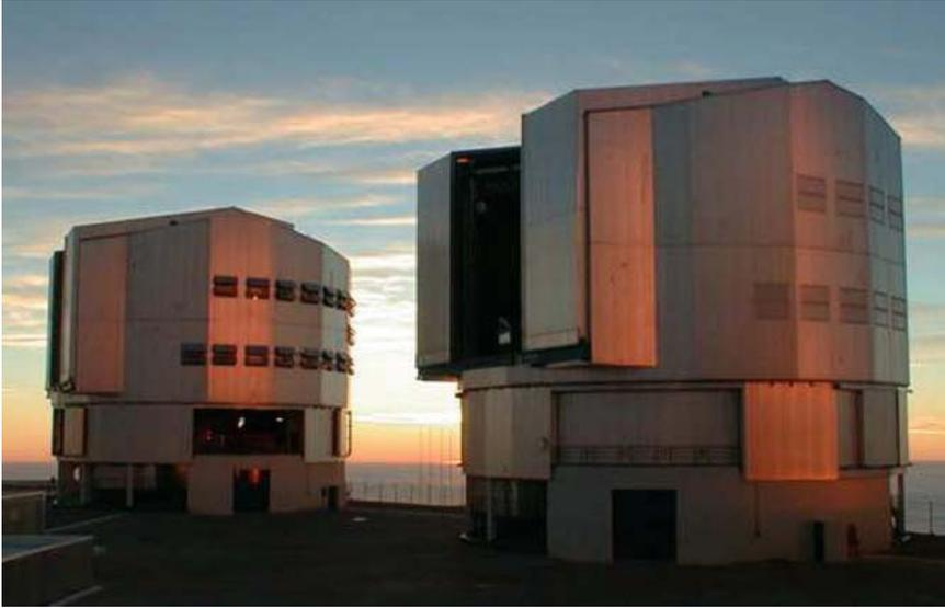
**Fig. 14.2** Very–Large–Telescope VLT (Paranal, Chile) with box–type enclosure and louvers for ventilation with ambient air [Courtesy ESO, Germany].
