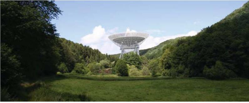
**Fig. 4.3a** View of the low altitude forested site Effelsberg, Germany (320 m altitude). The location in a valley provides wind protection [Courtesy N. Junkes, MPIfR, Germany].
