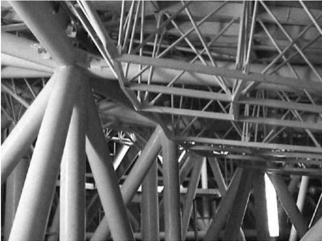
**Fig. 2.14** Partial view of the BUS tube network inside the IRAM 30-m telescope. Top of the figure: reflector side of the BUS. Big tubes: BUS network, smaller tubes of panel frames holding each 2 panels. The smaller tubes have a diameter of 2–3 cm [Courtesy J. Peñalver, IRAM, Spain].
