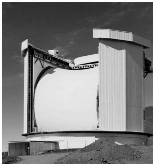
**Fig. 3.3** Astrodome of the 15-m James Clerk Maxwell Telescope (JCMT, Hawaii, USA, 4 000 m altitude). The astrodome consists of a steel housing that can be rotated. The ‘slit’ is covered by a membrane, it can be opened for special observations [Courtesy R.E. Hills, Cambridge, UK].
