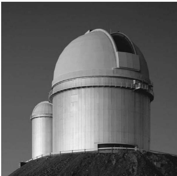
**Fig. 14.1** Conventional dome with slit of the ESO 3.6-m telescope (La Silla, Chile) [Courtesy ESO, Germany].
