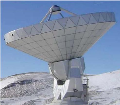
**Fig. 9.29.b** IRAM 15-m telescope of which the BUS is CLOSED by the panels and the rear cladding; the BUS network is protected against solar illumination and, to a large extent, against the thermal environment. An enclosed air volume can be ventilated/climatised.
