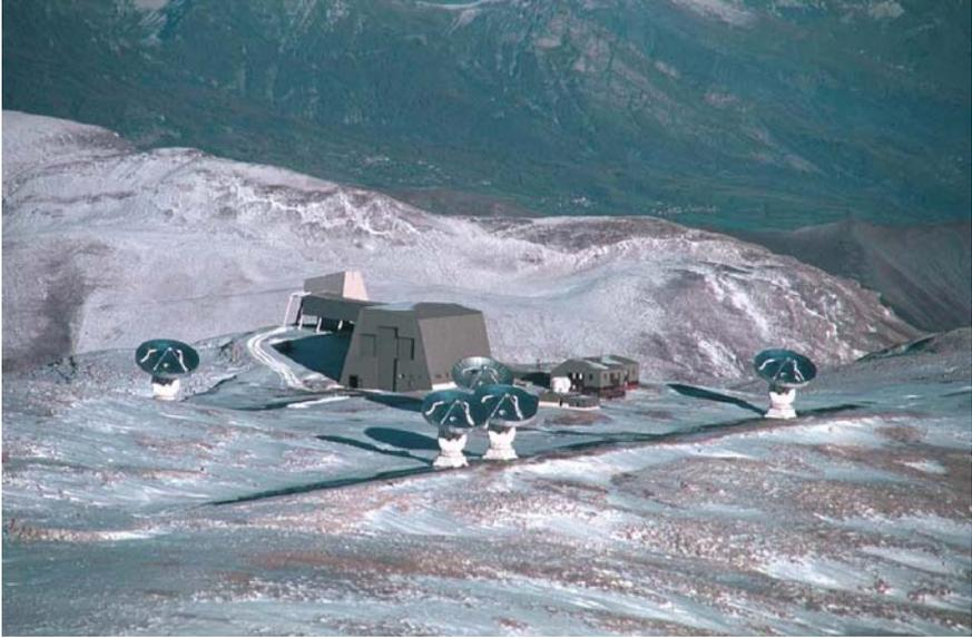
**Picture 1.7** Plateau de Bure Interferometer (French Alps, 2 500 m altitude). The telescopes can be displaced on the tracks (partially covered by snow) to form various interferometer configurations. At the centre of the observatory is a hangar that can house up to three telescopes for maintenance purposes [Courtesy IRAM, France].
