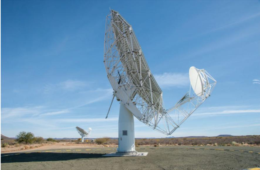
**Fig. 7.12** The first MeerKAT antenna of 13.5 m diameter in the Karoo desert of South Africa. The full array will contain 64 antennas spread over an area of 8 km diameter (J. Jonas, SKA-SA)
