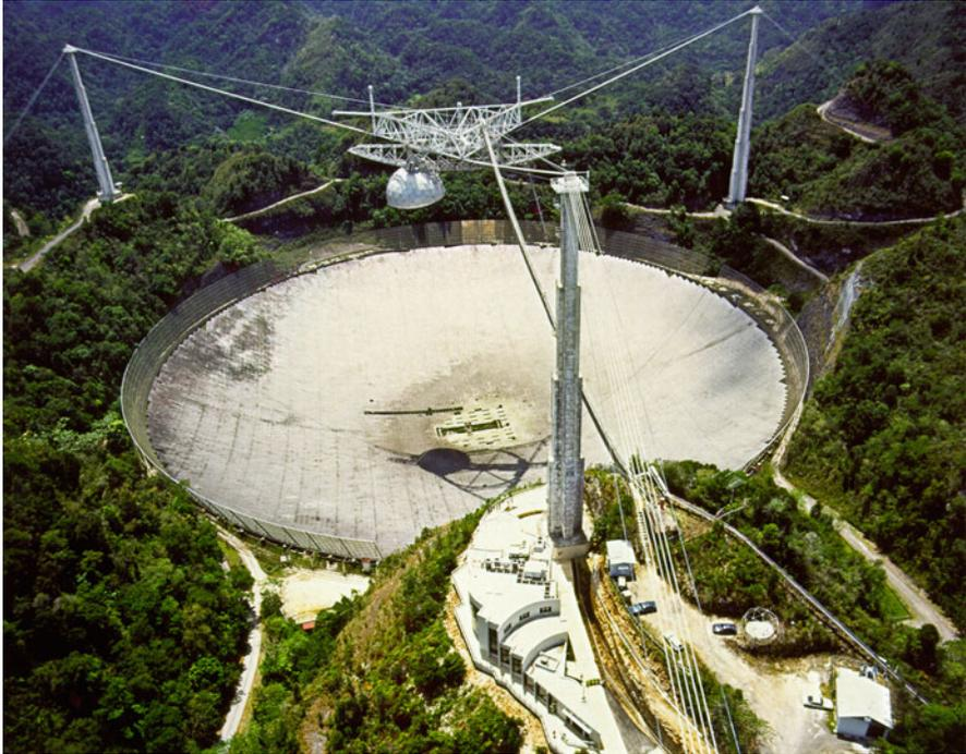
**Fig. 7.1** The 315-m diameter stationary, spherical Arecibo dish in Puerto Rico. The domed structure under the moving platform contains optics to create a point focus (NAIC—Arecibo Observatory, a facility of the NSF)
