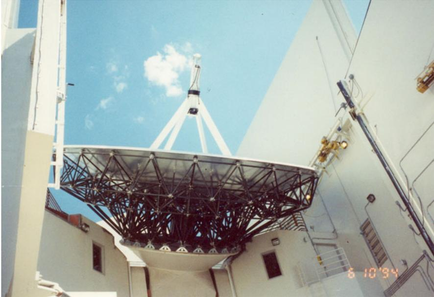
**Fig. 6.6** The quadripod, reflector and BUS attached to the upper flat plate of the mount. The antenna is placed in a protective enclosure. Here, the roof panels and doors are open for observations. The two dark windows in the building belong to the two instrument rooms with direct access to the Nasmyth focal points (J.Baars, SMT Observatory)
