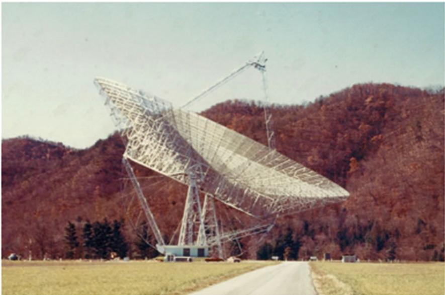
**Fig. 3.21** The original NRAO 300-ft transit telescope. The reflector structure is supported by two towers. The elevation drive is realised through a centre wheel with pinion and chain (J. Baars, NRAO/AUI/NSF)
