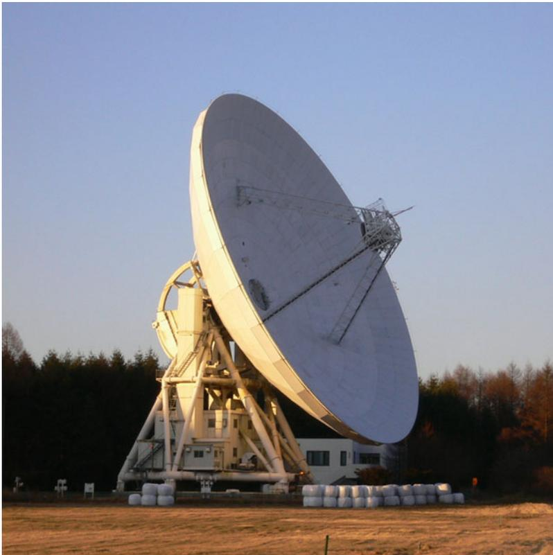
**Fig. 5.33** The 45-m diameter millimetre-wavelength telescope of the Nobeyama Observatory in Japan. It is the oldest large mm telescope (NRO/NAOJ)
