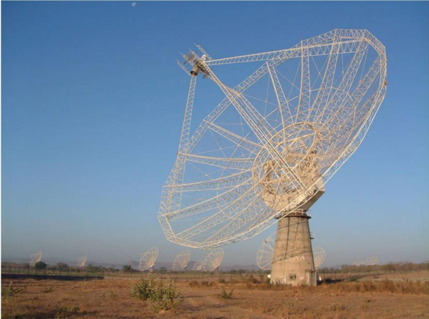
**Fig. 7.7** The GMRT array consists of 30 reflectors of 45 m diameter with a mesh surface. It operates from 38 to 420 MHz. The reflector is based on the SMART concept: Stretched Mesh Attached to Rope Trusses (Courtesy, G. Swarup, NCAR, India)
