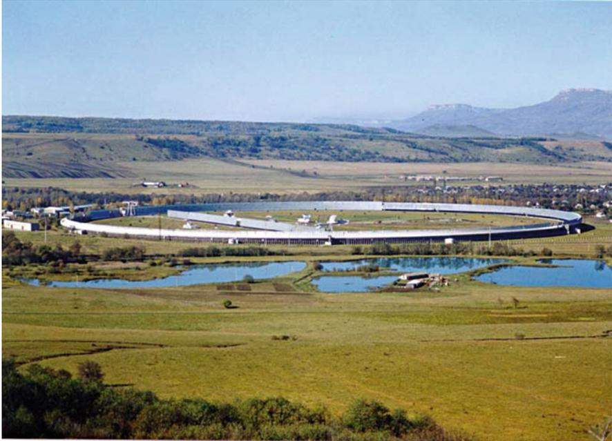
**Fig. 7.6** The 600-m diameter circular RATAN telescope. Several additional reflectors provide a number of different focal points. In the centre of the *circle* is a special reflector cone to concentrate the radiation onto a single horn feed. An angular resolution of 5 arcseconds can be achieved at the shortest wavelength of 1 cm (Special Astrophysical Observatory, Russia)
