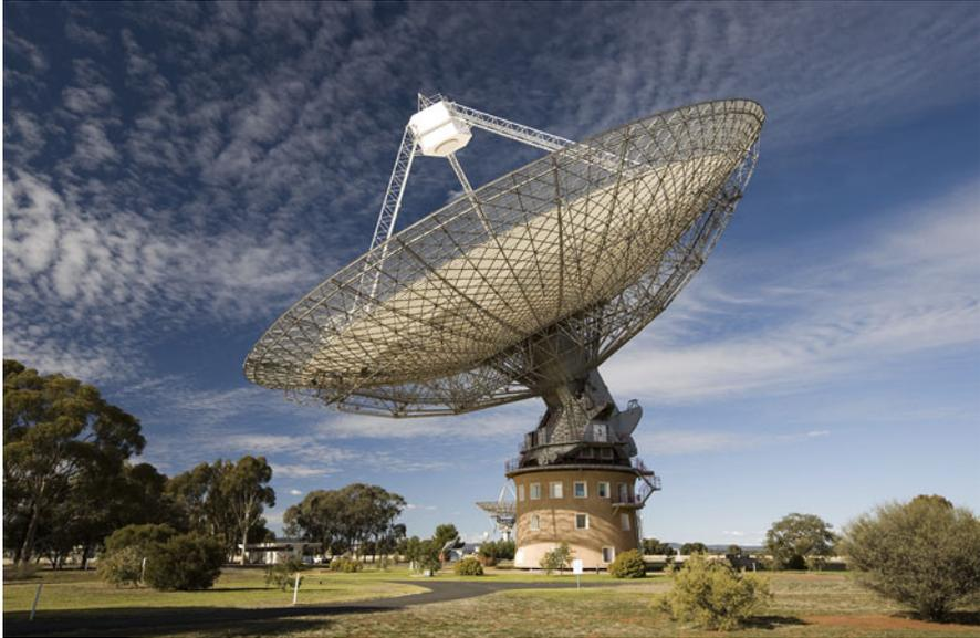
**Fig. 3.18** The Parkes telescope in its current situation with a partially closed surface and a larger focus cabin (CSIRO ATNF)
