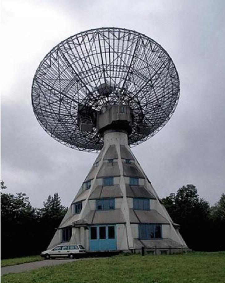
**Fig. 3.7** The Stockert 25-m radio telescope of the University of Bonn, Germany, employs a compact “king-post” mount design for the axes movements. Also here originally a central mast for the feed was used; it was later replaced by a subreflector to form a Cassegrain configuration (Astron. Inst. Univ. Bonn)
