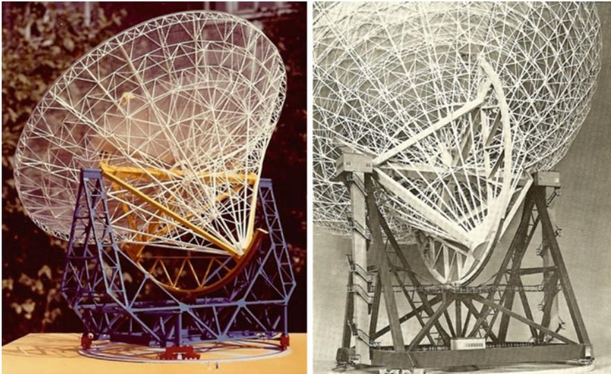
**Fig. 4.10** Models of the Krupp design for an 80-m telescope with separate elevation cradle. First proposal on the *left* and final design on the *right* (Krupp)
