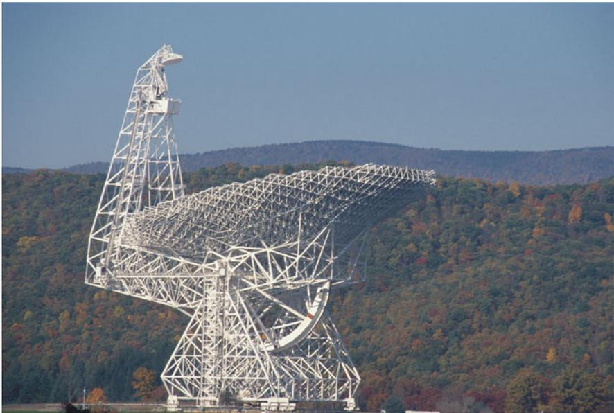
**Fig. 7.14** The Green Bank Telescope (GBT) with an effective diameter of 100 m. The Gregorian optics enables operation from both the primary and secondary focus (NRAO/AUI/NSF)
