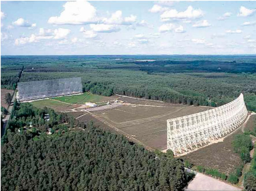
**Fig. 7.5** The Nançay Radio Observatory Kraus-type telescope with fixed spherical reflector (*right*), which reflects the radiation coming from the flat, tilttable reflector at *left* to the focal area near the ground in front of the flat (*white cabin*) (Nançay Radio Observatory, France)
