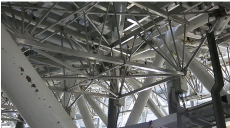
Fig. 5.30 Rear view of the installed panel segments inside the backup truss
