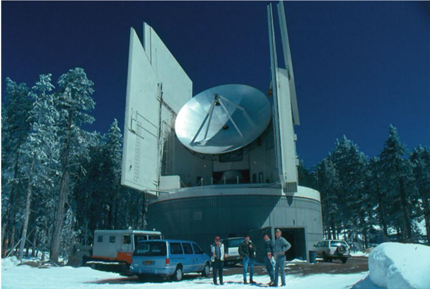
**Fig. 6.7** The HHT in the opened protective enclosure. The hydraulically powered roof and door panels are closed during inclement weather (J.Baars, SMT Observatory)
