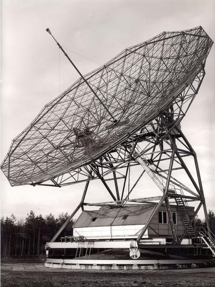
**Fig. 3.5** The Dwingeloo 25-m radio telescope in the Netherlands was the biggest in the world for about a year, when the 76-m Jodrell Bank telescope overtook it. The alt-azimuth design employs a “wheel on track” for the azimuth movement. The central mast carries the dipole feed in the focal point and a small receiver package behind the focus (ASTRON)
