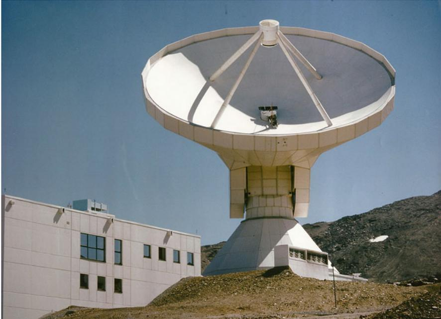
**Fig. 5.5** The MRT is covered on the outside with thermal insulation. The skin of the cladding can be heated to avoid ice deposit. The extended rim at the top of the reflector avoids ice or snow to fall onto the reflector surface (IRAM)
