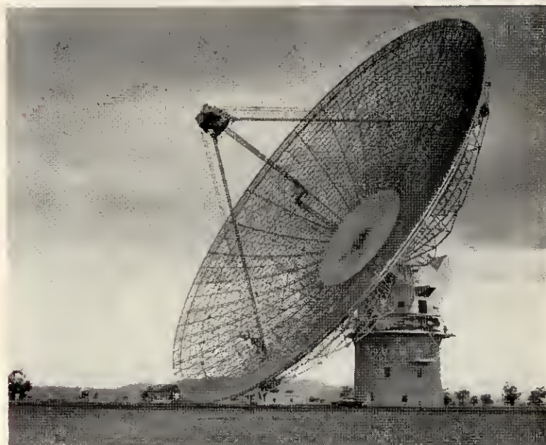
Plate II. Recently-completed 210-foot-diameter parabolic radio telescope of the Commonwealth Scientific and Industrial Research Organization in Australia. (Photograph courtesy of C.S.I.R.O. Radiophysics Laboratory.)
