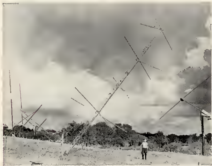
Plate IV. A crossed-yagi parabolimeter antenna at the University of Florida Radio Observatory.
