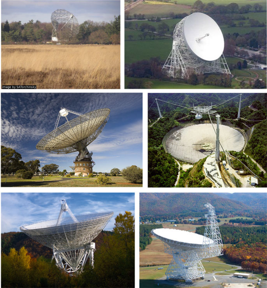
Fig. 1.3 Classic single-dish radio telescopes. Top left: Dwingeloo 25 m telescope (Netherlands ca. 1956, photo © Steve Torchinsky); Top right: Jodrell Bank 76 m Lovell telescope (UK ca. 1957, photo © Cavendish); Middle left: Parkes 64 m telescope (Australia ca. 1961, photo © CSIRO); Middle right: Arecibo 300 m telescope (US ca. 1963, photo © NAIC/NSF); Bottom left: Effelsberg 100 m telescope (Germany ca. 1972, photo © MPIfR); Bottom right: Green Bank Telescope (US ca. 2000, photo © NRAO)
