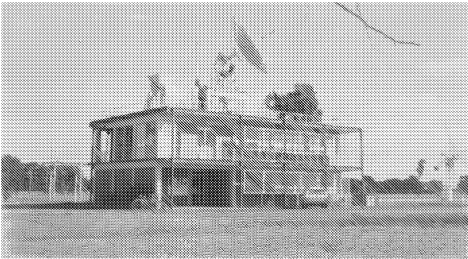
Plate B: The central Culgoora observatory building which houses the radioheliograph and radio-spectrograph equipments. (Courtesy of J. P. Wild and K. V. Sheridan).
