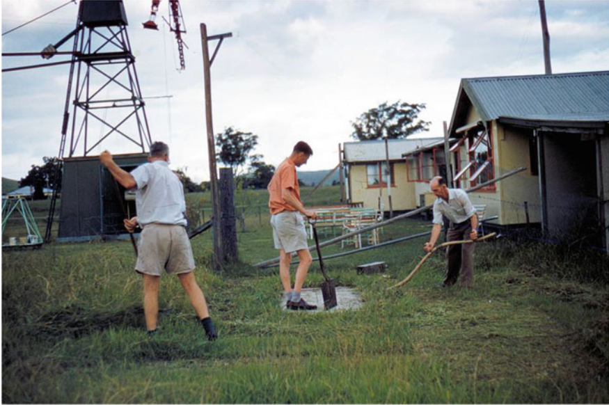
Fig. 5.8 Paul ( centre ) and Kevin Sheridan ( right ) doing maintenance work at the Dapto field station (CSIRO Radio Astronomy Historical Photographic Archives P13114-9)
