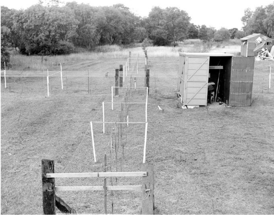
Fig. 3.7 A close-up view of the prototype Mills Cross at the Potts Hill field station. The prototype cross operated at 97 MHz with a beamwidth of 8^\circ . Each arm of the cross was 36 m in length (Courtesy of CSIRO Radio Astronomy Image Archive: B3064-3 Image Date: 21 April 1953)
