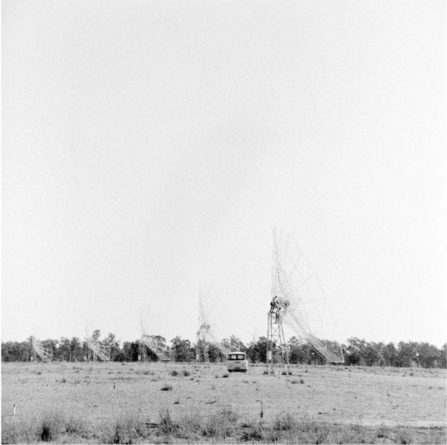
Fig. 5.27 The radioheliograph aerials following assembly on their mounts (CSIRO Radio Astronomy Historical Photographic Archives B7515-26)
