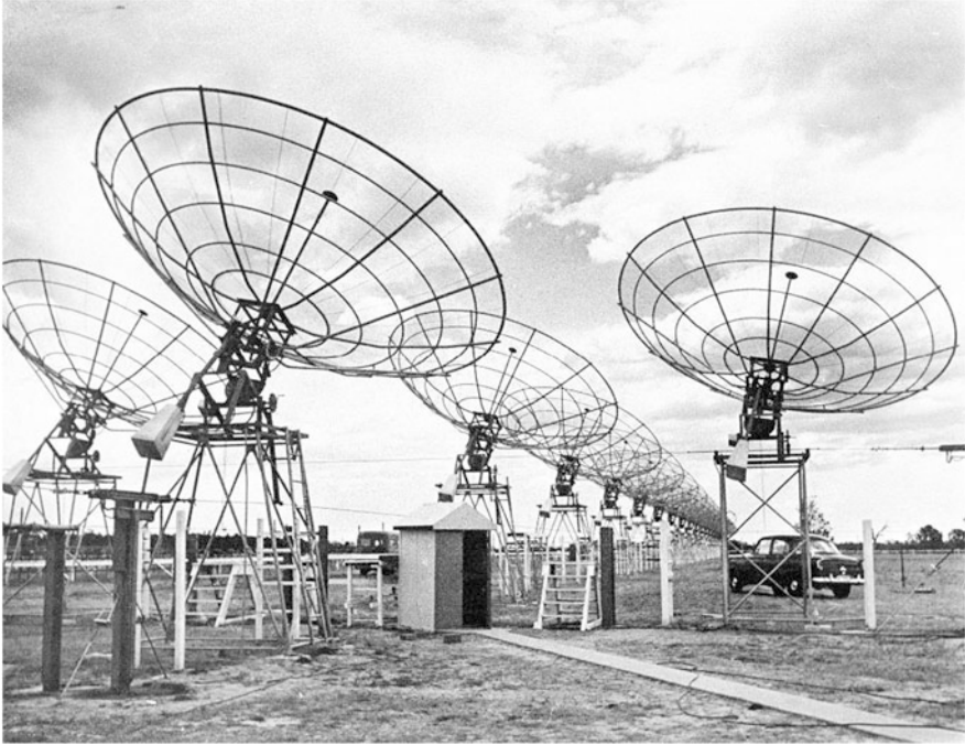
Fig. 4.17 The completed Chris Cross at Fleurs field station in November 1957. The view is from just north of the centre of the array looking south along the N-S arm. Each arm had 32 5.8 m open mesh dishes operating at 1420 MHz and producing a 3 arcmin pencil beam (CSIRO Radio Astronomy Historical Photographic Archives B5219-2)
