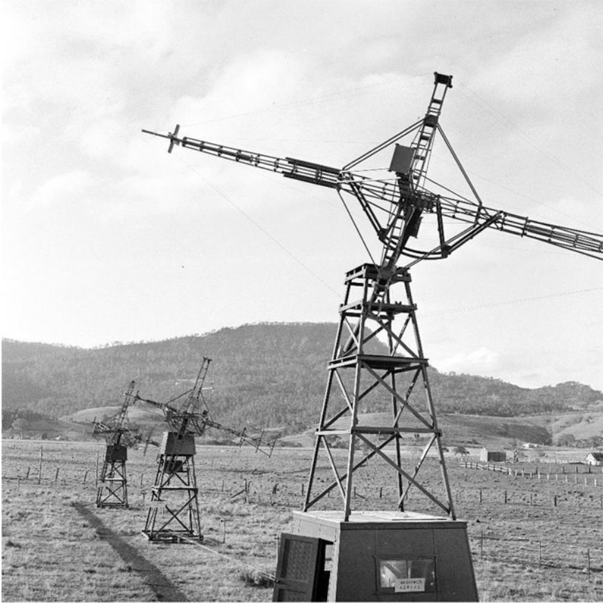
Fig. 5.7 The three completed cross-rhombic aerials of the solar spectrograph at Dapto field station in September 1952 (CSIRO Radio Astronomy Historical Photographic Archives B2888-2)
