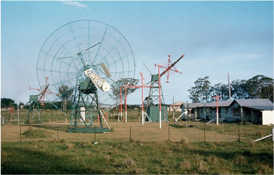
Fig. 5.17 Dapto field station showing the 200–2000 MHz parabolic aerial together with the three original rhombic aerials (CSIRO Radio Astronomy Historical Photographic Archives P10478-2)
