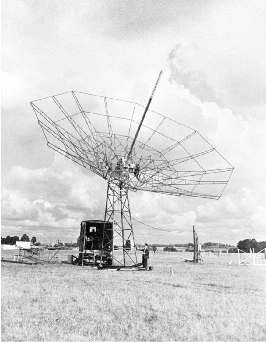
Fig. 5.24 A full-scale prototype of one of the radioheliograph aerials undergoing testing in 1963 (CSIRO Radio Astronomy Historical Photographic Archives B7268-2)
