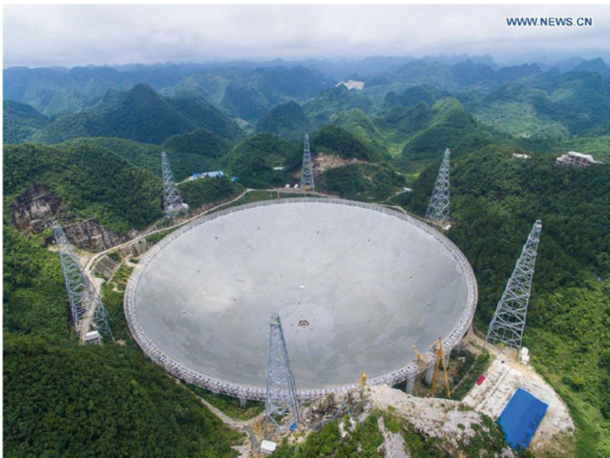
Fig. A.3 The Five-hundred-metre Aperture Spherical Telescope (FAST) in China. The receiver is suspended at the prime focus point by cables from the surrounding towers. It began observations in September 2016 (Credit Xinhau)
