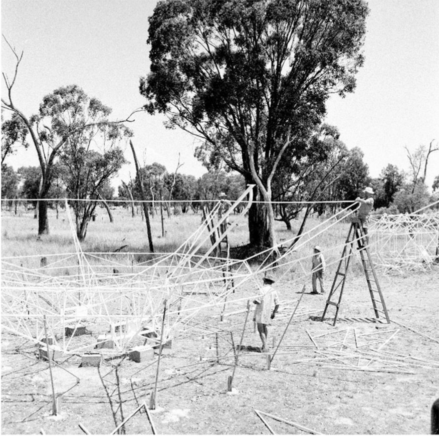
Fig. 5.25 Fabricating one of the 96 aerials of the radioheliograph on site at Culgoora in 1964 (CSIRO Radio Astronomy Historical Photographic Archives B7354-10)
