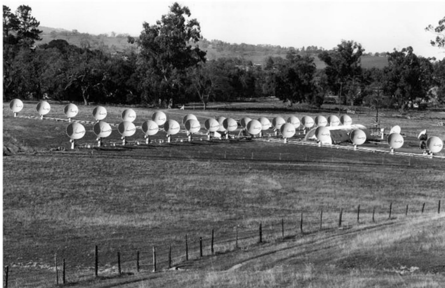
Fig. 6.8 The crossed-grating array named the Stanford Microwave Spectroheliograph. The array operated at a wavelength of 9.1 cm and was used to produce daily two-dimensional maps of the sun with a resolution of 3.2 min of arc from June 1962 until August 1973. The observatory was named “Heliopolis” by Bracewell (Courtesy of the Goss Collection)
