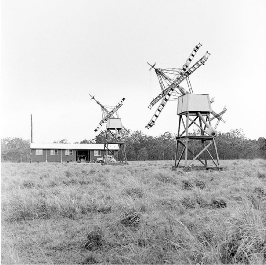
Fig. 5.6 Two of the three crossed-rhombic aerials in final stages of construction at Dapto field station, near Wollongong in November 1951. Each aerial is equatorially mounted to track the sun and operated in three bands, 40–75, 75–140 and 140–240 MHz. In the background is the receiver hut. The spectrographs became operational in August of 1952 (CSIRO Radio Astronomy Historical Photographic Archives B2640-5)
