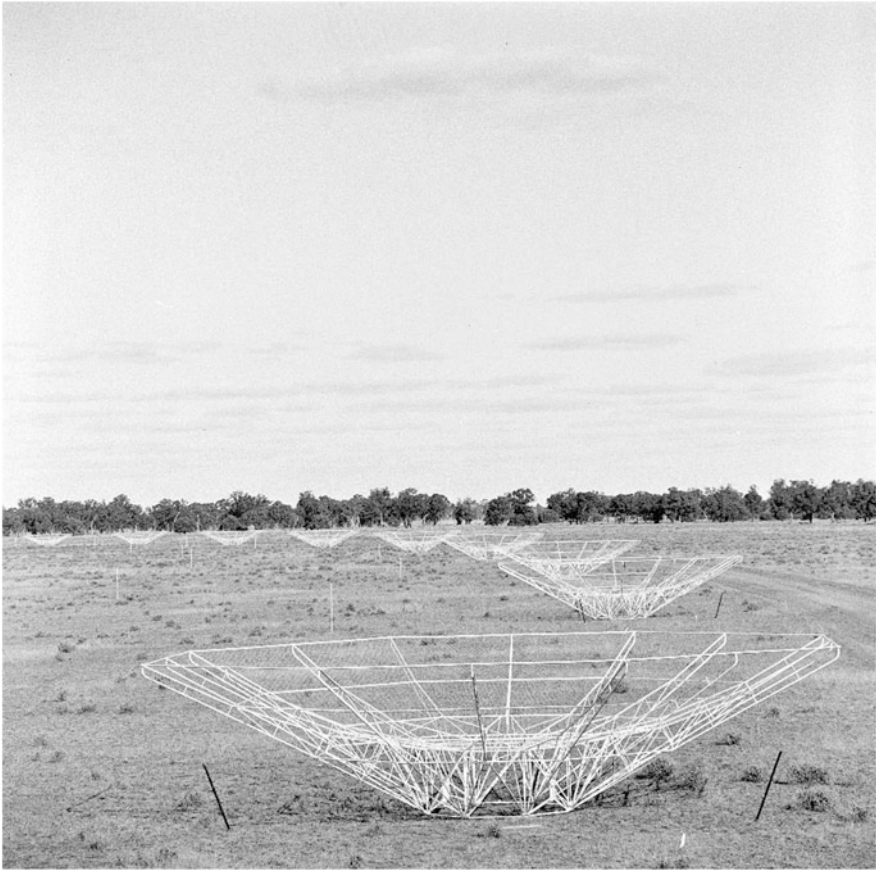
Fig. 5.26 The radioheliograph aerials laid out ready for mounting at Culgoora in 1964 (CSIRO Radio Astronomy Historical Photographic Archives B7515-22)
