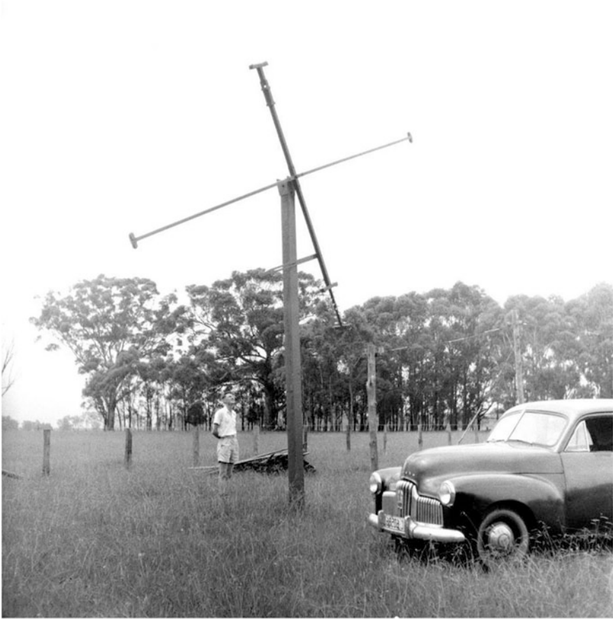
Fig. 5.12 Wild standing next to one of the swept-frequency interferometer rhombic aerials at Dapto field station in March 1955. The open wire transmission lines are visible on the post on the right on the image. Two aerials were arranged on an east-west baseline 1 km apart, with a second pair of aerials at a shorter baseline of 0.25 km used to assist in accurate lobe identification. In the late 1950s, the swept-frequency interferometer was extended to a swept-lobe interferometer (CSIRO Radio Astronomy Historical Photographic Archives 3590-2)
