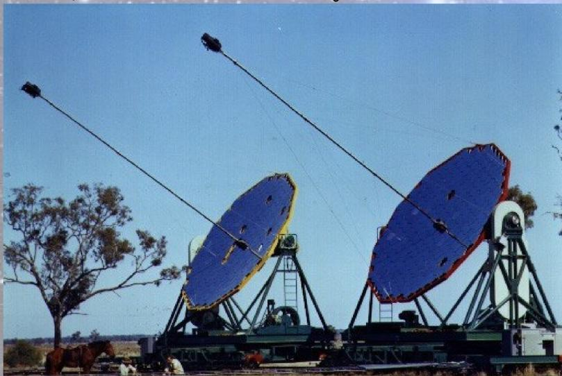
Figure 8: The Narrabri Intensity Interferometer was constructed in 1965 and operated until 1971. Each telescope was 6m in diameter, twice as large as the StarBase telescopes.
