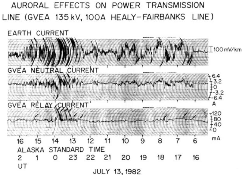
Figure 6.13 From the top, the Earth current recorded at the Geophysical Institute, University of Alaska, electric currents induced in the Golden Valley Electric Association (GVEA) power transmission line and the relay current in the GVEA substation on July 19, 1982: S.-I. Akasofu and J. Aspnes (1982).
