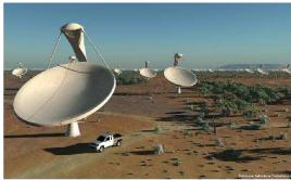
**FIGURE 10.** Planned SKA configurations: dipoles for low frequencies (70–450 MHz) (left) and dishes for high frequencies (450 MHz–3 GHz) (Copyright: Swinburne Astronomy Productions and SKA Project Development Office).
