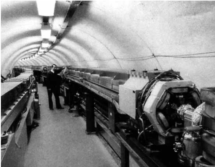
Inside the tunnel, circa 1983. (Cornell 2000)
