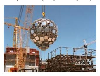
**Fig. 1.** Sphere of 10 m diameter at the NIF laser at the Lawrence Livermore National Laboratory LLNL in California where Laser beams are irradiated into the holes to and focused to diameters of about 100 micrometer diameter into holes of a capsule for indirect drive DT fusion in a sphere with a diameter above one millimeter producing the highest nuclear fusion gains (Hurricane *et al.*, 2014; Hinkel *et al.*, 2016).
