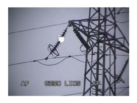
Example: a UV image of the HV corona discharge obtained with image intensifies combined with a narrow band filters. During the day time this corona is practically undetectable in the visible region of spectra
