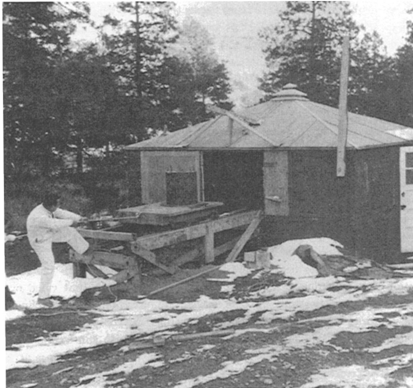
Fig. 14.1. "Remote handling" of a kilocurie source of radiolanthanum for RaLa testing. LA Photo, 26406.
