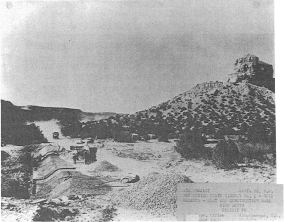
Fig. 4.4. New Mexico State Highway No. 4, the first major road built leading to Los Alamos, October 1943. LA Photo, 00384.
