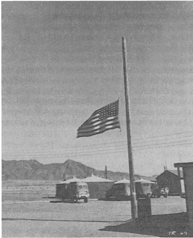
Fig. 18.1. Base camp, completed in December 1944, was the main service area for the Trinity Test in July 1945. LA Photo, TR49.
