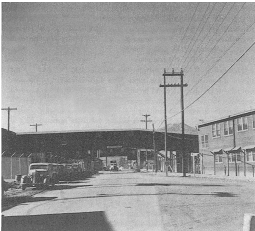
Fig. 16.1. Covered passage over Los Alamos main road. Building P, housing the experimental physics division, is on the left. Building T, housing the theoretical physics division, is on the right, partially hidden by the bridge. LA Photo, 3736.
