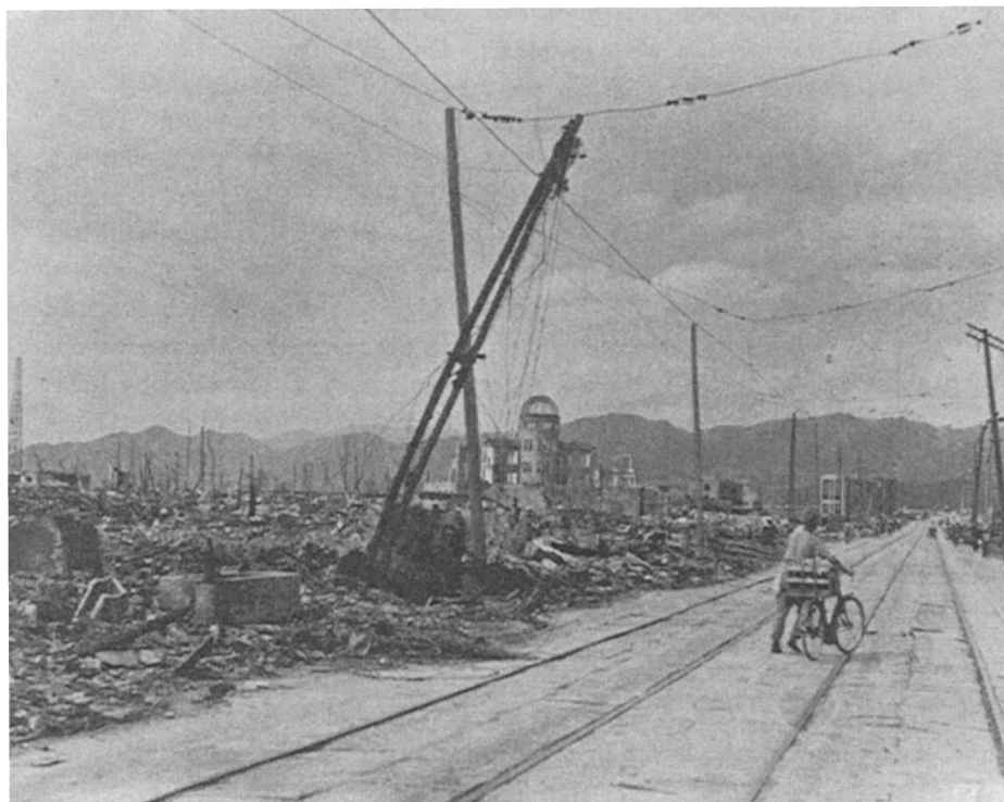
Fig. 19.4. View of Hiroshima city after Little Boy was dropped. LA Photo, TR 720.
