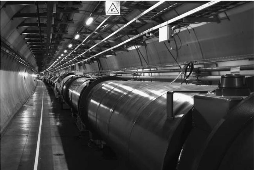
**Figure 6.2** Dipole magnets installed inside the LHC tunnel.
