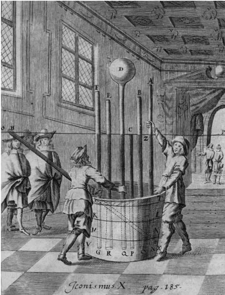
**Figure 8.6** Torricelli's experiment disproving *horror vacui*: the columns of mercury fall at the same height in all containers, independently of the volume left empty.
