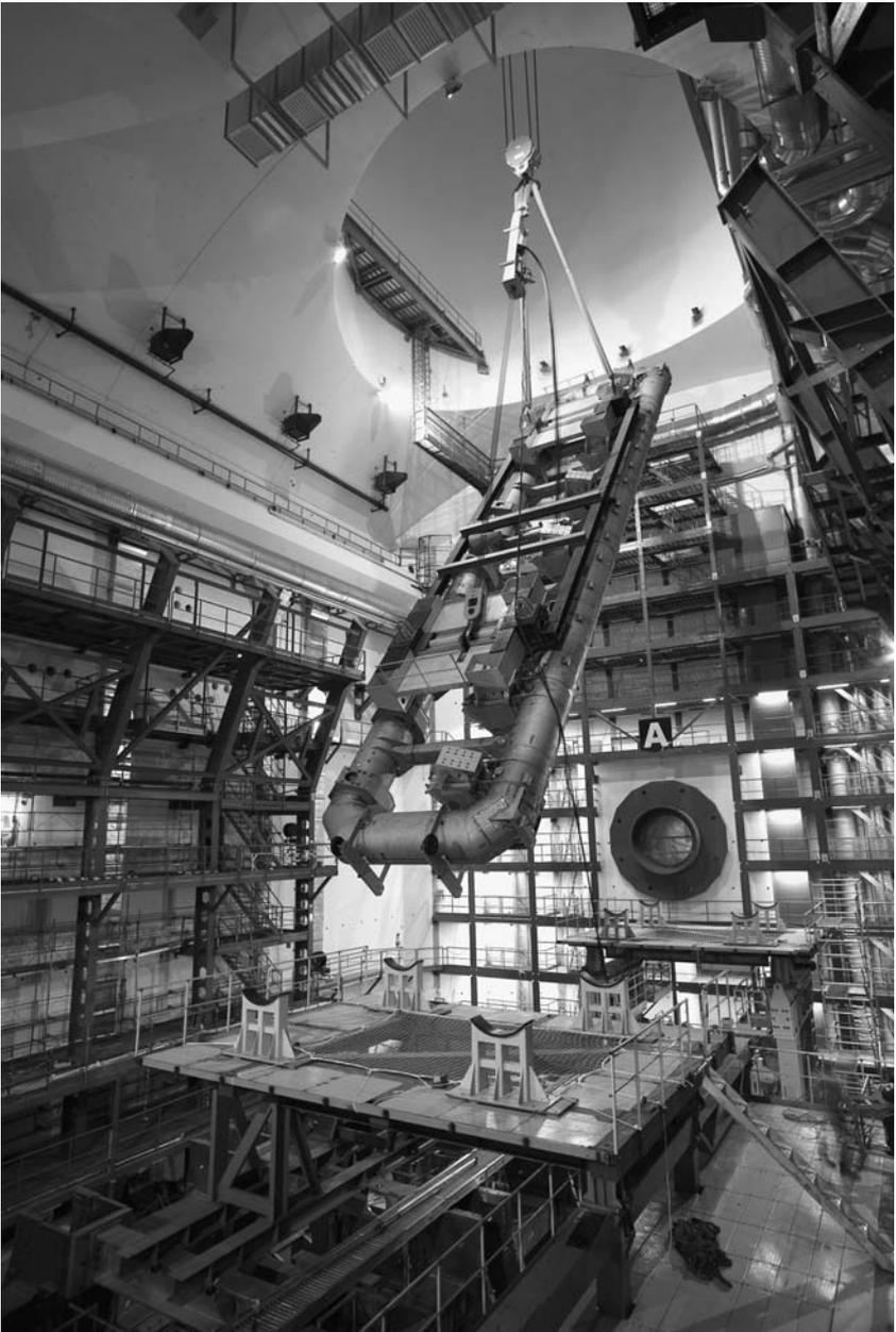
**Figure 7.8** Descent of the first superconducting coil inside the ATLAS cavern on 26 October 2004.
