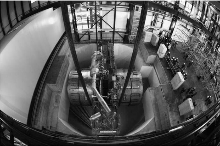
**Figure 7.10** Lowering of the heaviest piece of the CMS detector on 28 February 2007.
