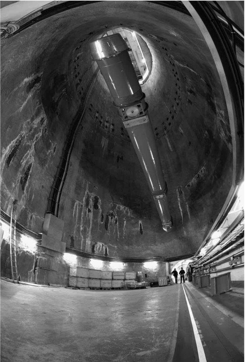
**Figure 6.5** Descent of an LHC dipole into the tunnel.
