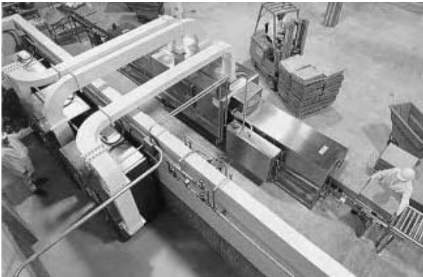
Fig. 6.1 Tempering tunnel (Defreeze Corporation).
