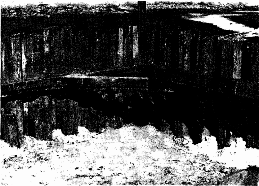
Fig. 10-4 Steel Sheet Pile CutOff (Guertin, 1982)
