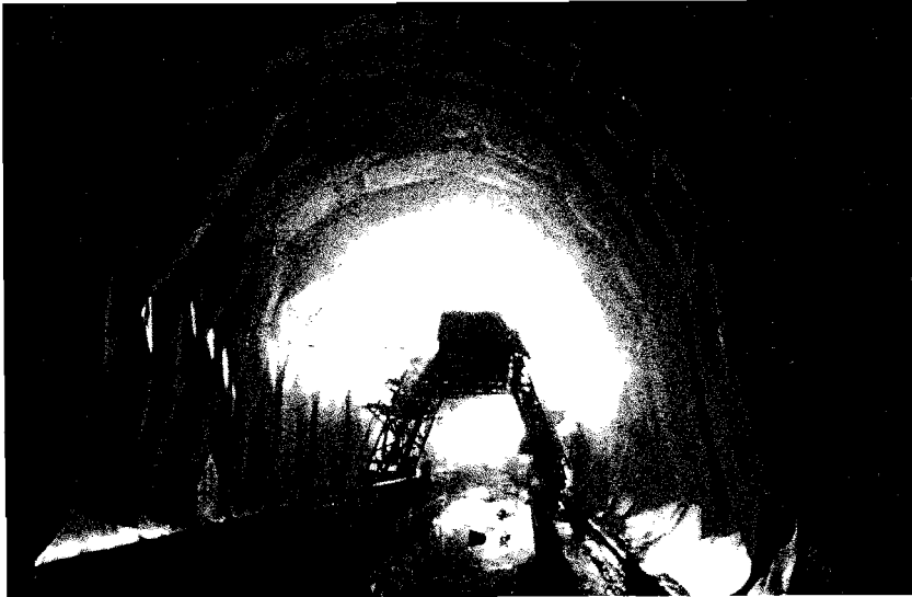
Fig. 10-22 Tunnel Membrane in Place, Washington, D.C. (Strasser, 1988)
