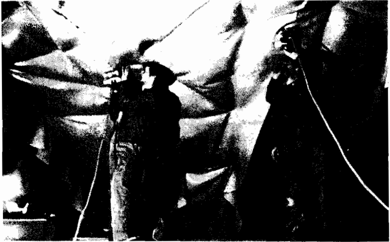
Fig. 10-17 Thermal Welding Waterproofing Sheet (Gnilsen, 1986)
