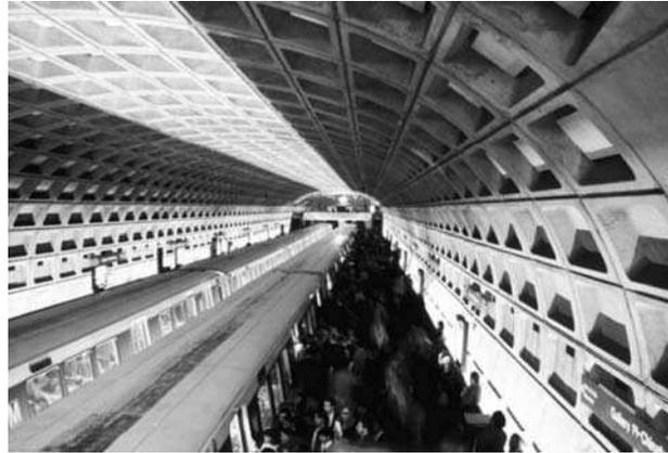
Fig. 17.1 Precast lining in a metro tunnel (Ref: <http://www.railwayage.com/sept01/washmetro.html>).
