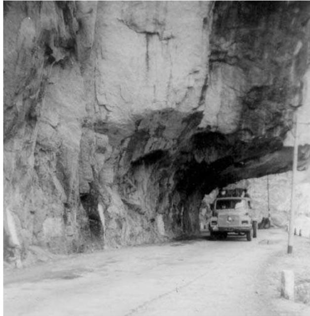
Fig. 25.1 Photograph of a half tunnel (Anbalagan et al., 2003).
