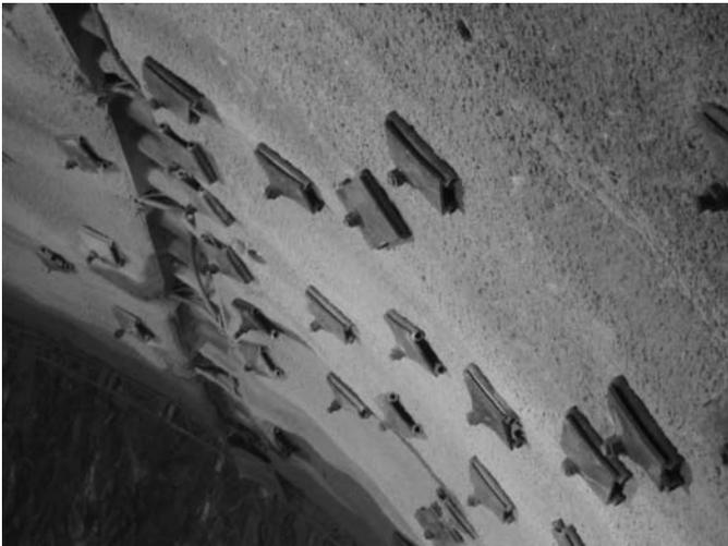
**Fig. 14.29.** Anchor headplates and pipe array
