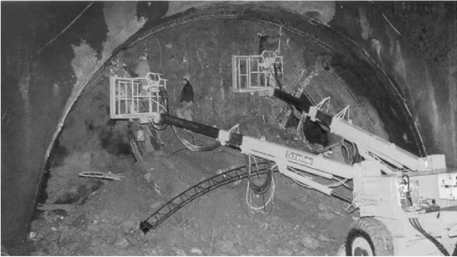
**Fig. 5.24.** Mounting of girder arches, Zürich-Thalwil tunnel<sup>17</sup>
