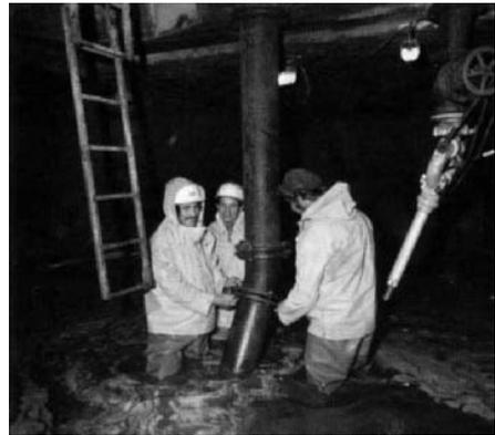
**Fig. 10.4.** Work chamber of a pneumatic caisson (Metro Amsterdam)
