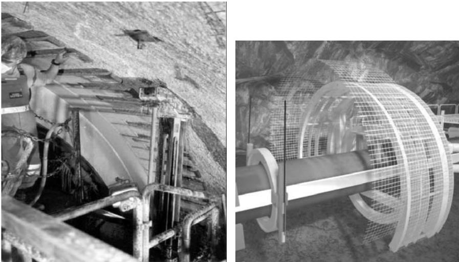
**Fig. 4.13.** left: Anchoring behind the cutterhead; right: Installation of wire mesh behind the cutterhead<sup>10</sup>
