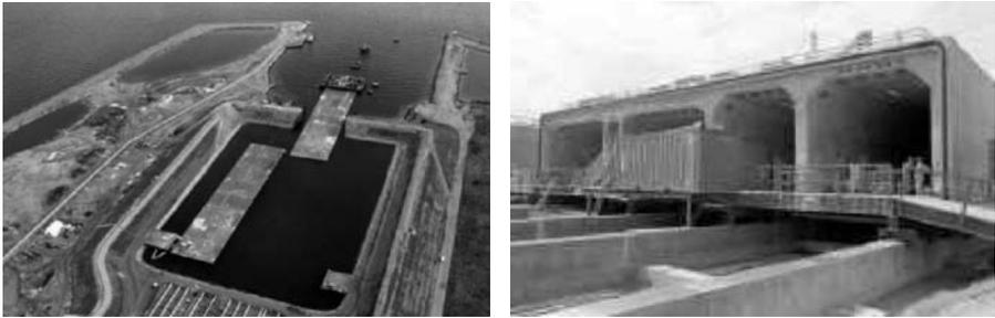
Fig. 10.2. Pre-fabricated tunnel blocks for Øresund tunnel<sup>4</sup>
