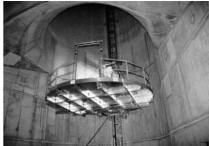
**Fig. 11.3.** *Alimak* - lift platform
