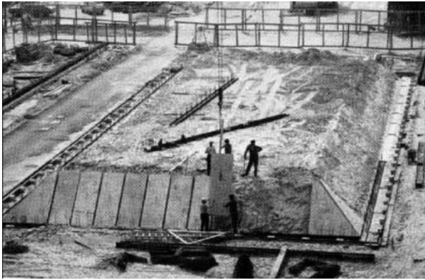
**Fig. 10.5.** Caisson for Metro Amsterdam: mould for concrete
