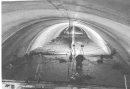
**Fig. 2.6.** Supply and extract channels above the carriageway. The separating vertical wall has not yet been mounted.<sup>14</sup>
