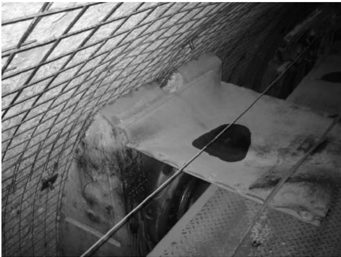
**Fig. 5.5.** Shotcrete hood in TBM heading of Loetschberg base tunnel
