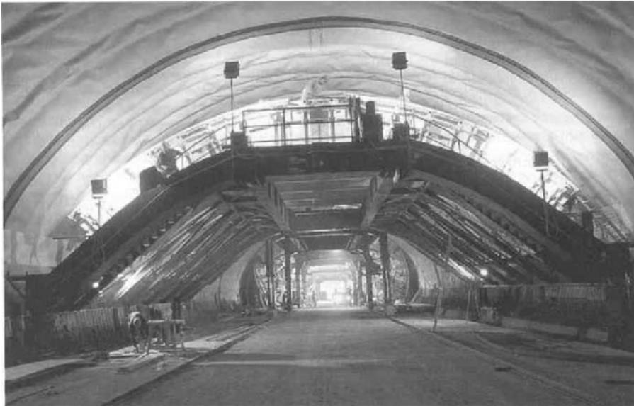
**Fig. 5.30.** Rolling formwork (Engelberg base tunnel)<sup>26</sup>
