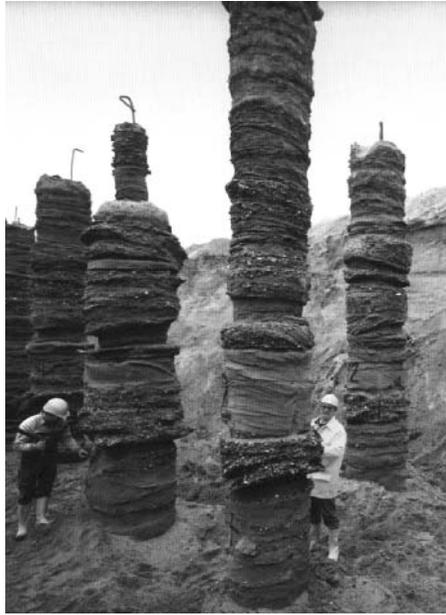
**Fig. 6.5.** Uncovered jet-grout columns produced in layered soil<sup>4</sup>
