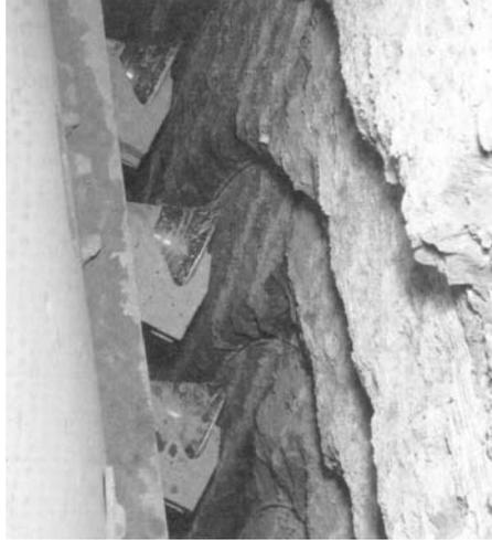
Fig. 4.63. Undercutting at the Uetliberg tunnel<sup>58</sup>
