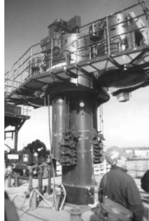
**Fig. 10.3.** Pneumatic caisson, lock (right)
