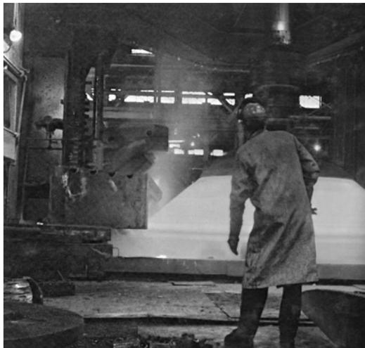
**FIGURE 2.12** Forming a formed head in the mill.
