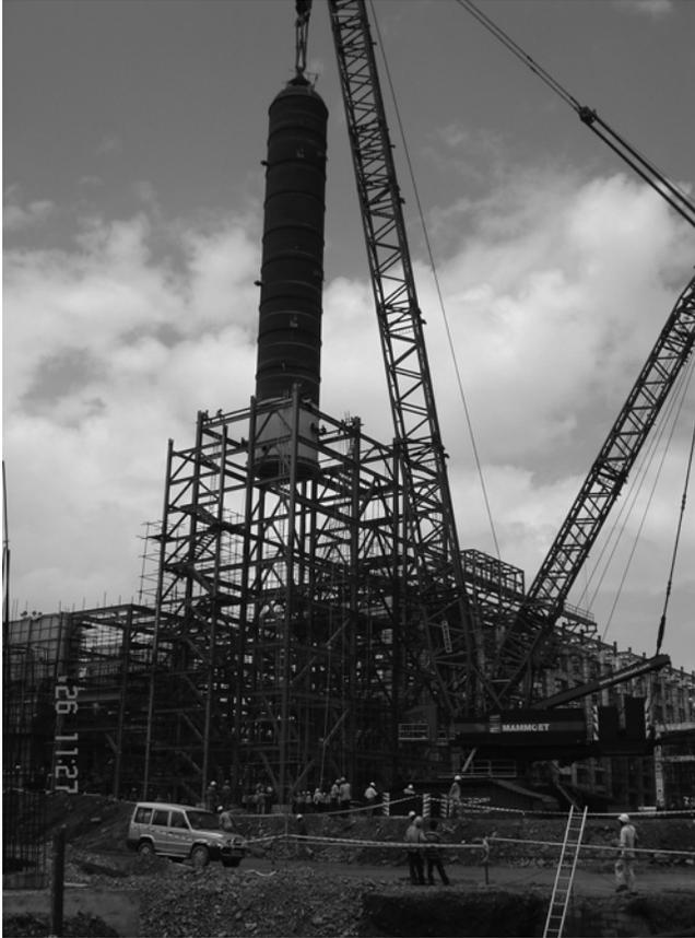
**FIGURE 7.23** The lowering and final installation of the hydrocracker referred to in [Figure 7.22](#).
