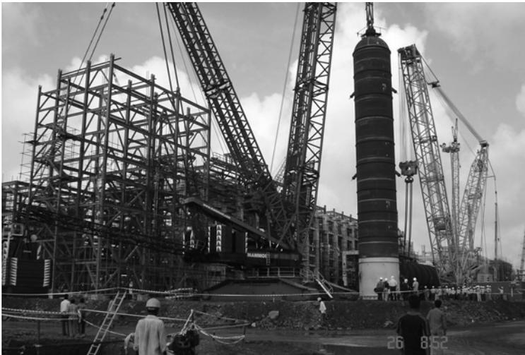
**FIGURE 7.22** The actual lifting of the hydrocracker using the top flange lug and tail lugs.
