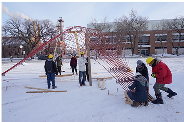
Figure 1. Students assembling the bending active framed vault (photo by Dominique Rey and Lancelot Coar).
