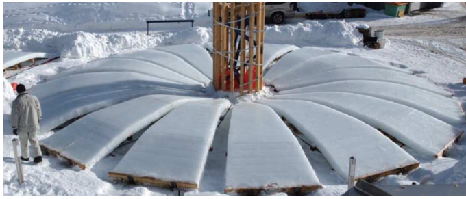
Figure 2. Segmented ice dome in Austria; ice segments during the creeping process (Dallinger & Kollegger 2012).
