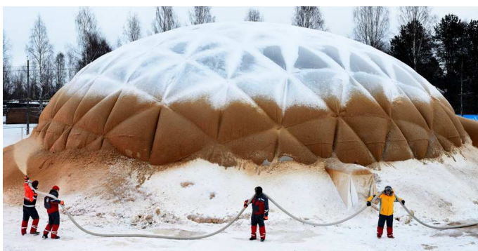
Figure 3. Spraying of wood fibre-ice composite in Finland, winter of 2013/2014 (photo: B. van Overbeeke, TUE).
