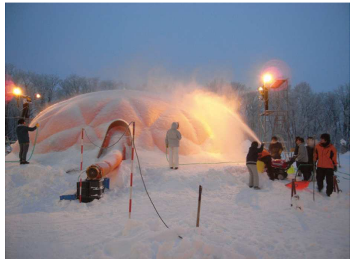
Figure 1. Application of snow and water on pneumatic formwork to create a spherical dome in Japan (Kokawa et al. 2012).
