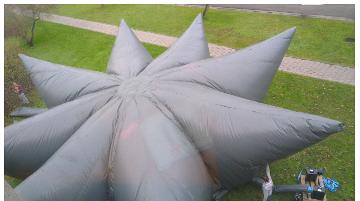
Figure 6. Test inflation of the fabric formwork for the Candela pavilion at Ghent University during the fall of 2015.
