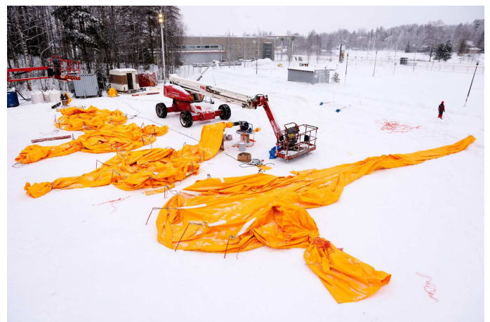
Figure 4. Formwork fabric for the four front towers of the Sagrada Familia project ready to be inflated (Photo: Bart van Overbeeke, TUE).
