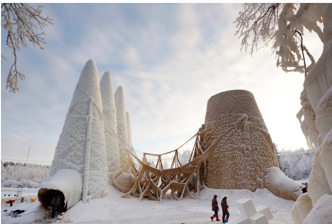
Figure 5. Wood fibre-ice composite church, with four front towers, column-suspended branching cables for the ship, and unfinished main tower, winter 2014/2015 (photo: Bart van Overbeeke, Tue)
