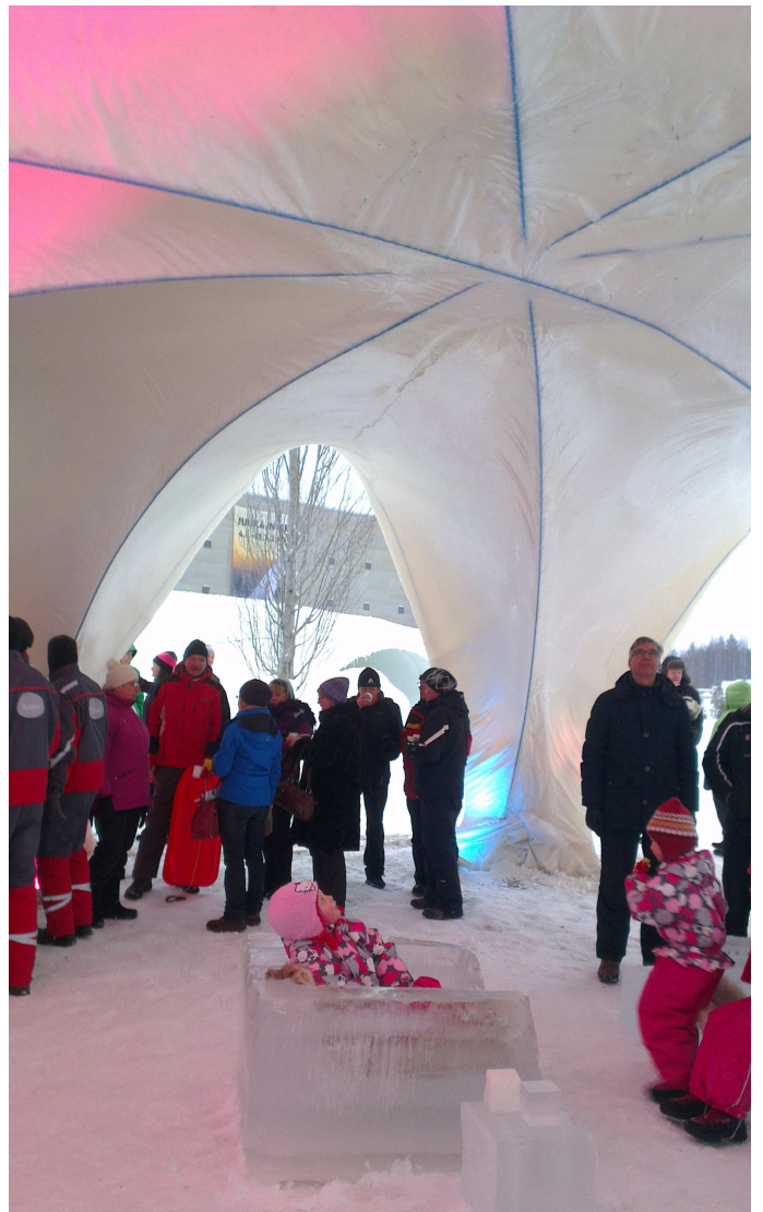
Figure 9. Interior of the Candela pavilion in cellulose-ice composite with blue articulated ropes used to preload the inflatable formwork.
