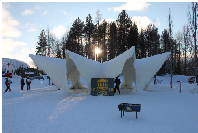
Figure 7. Candela Pavilion after removal of the balloon, before cutting of the edges.
