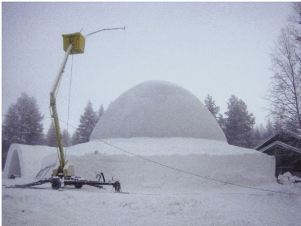
Image 4. Oval three-layer structure under construction (Ryynänen 2011)
