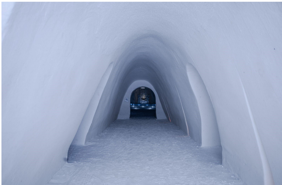
Image 9. Arc-shaped snow corridor (Pernu 2024)
