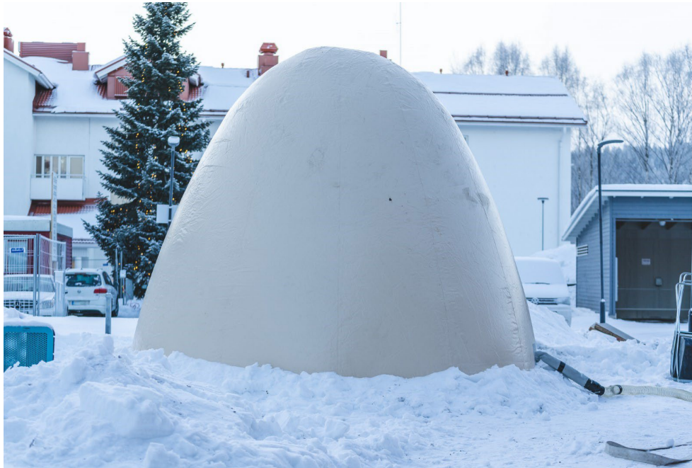
Image 7. A catenary-shaped air pressure mould (Pernu 2022)
