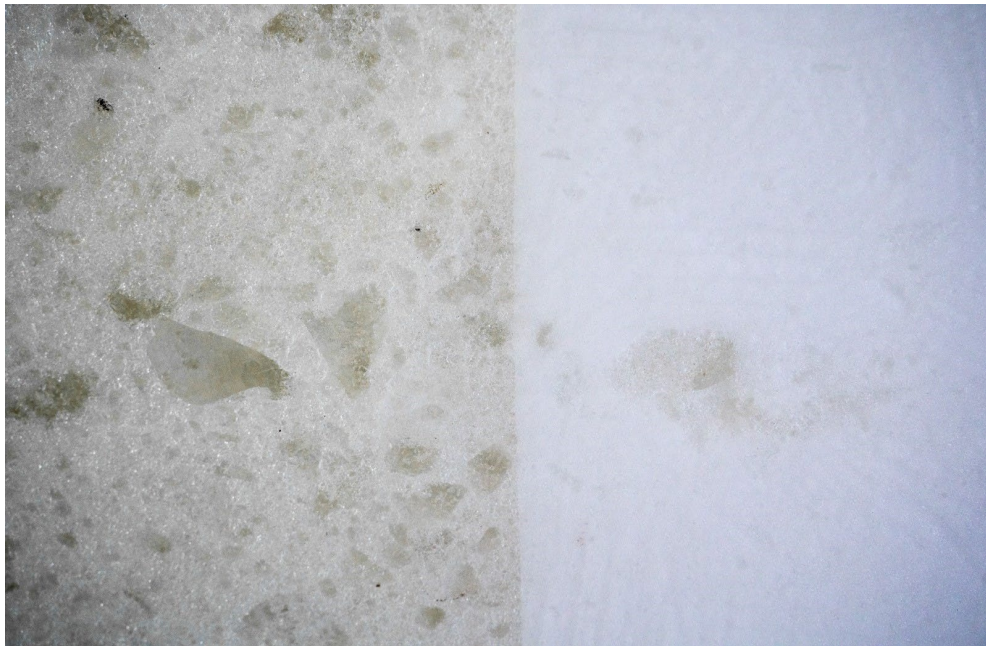
Image 16. Stored snow and ice (left) and fresh snow (right) in a single structure at the Lehtojärvi snow and ice hotel (Pernu 2025)
