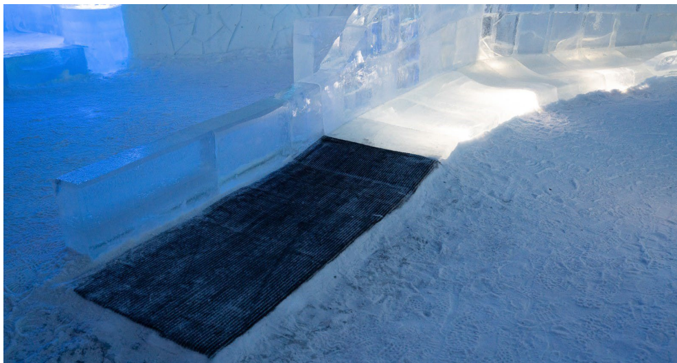
Image 31. A rubber mat placed at the end of a slide to stop users (Pernu 2024)
