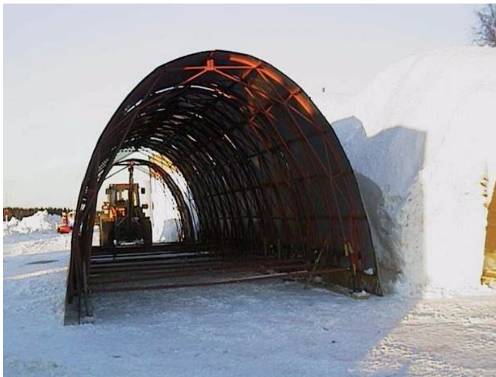
Image 6. Steel catenary-shaped vault mould (Ryynänen 2011)
