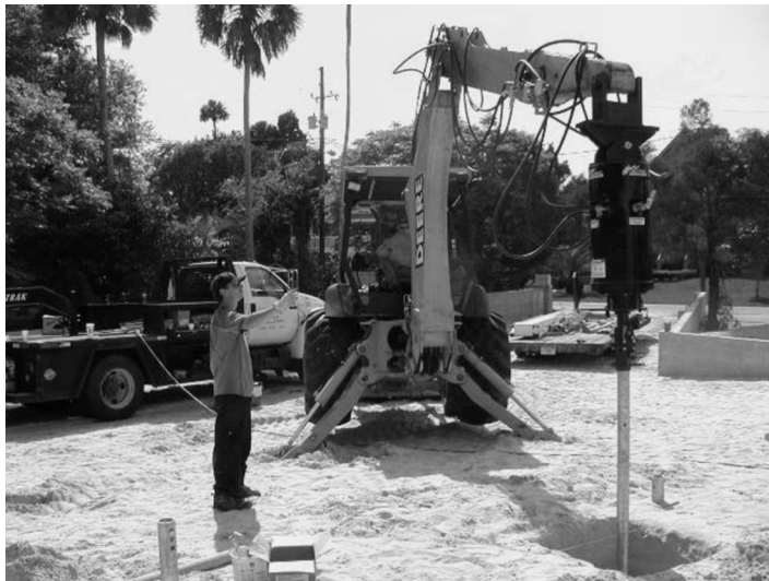
Figure 12.3 Installation of residential foundation (Courtesy of ECP)
