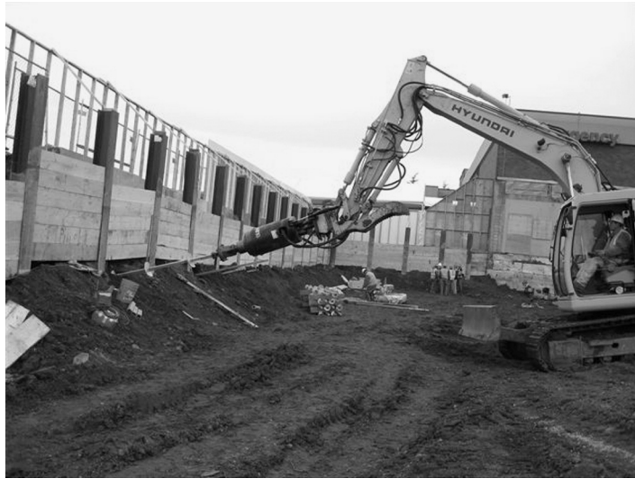
Figure 13.12 Installation of helical anchor for soldier pile and lagging system (Courtesy of ECP)
