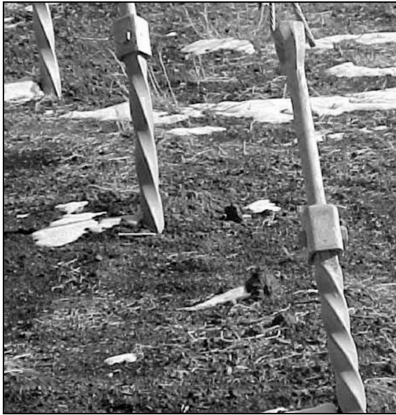
Figure 2.23 Twisted helical anchor shafts (Downey, 2008)
