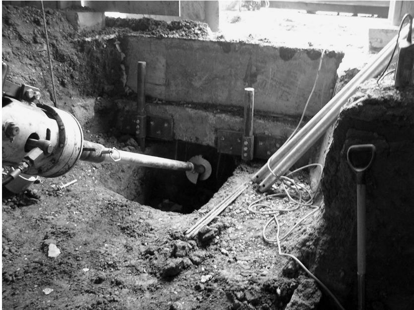
Figure 14.10 Installation of Top Row Helical Anchors (Stage 1)
