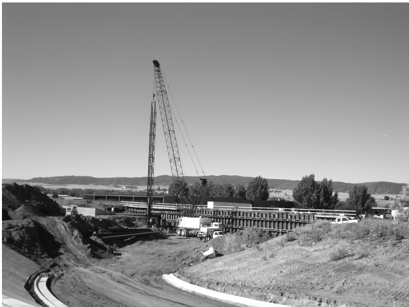
Figure 13.10 Sheet pile and helical anchor wall (Courtesy of Magnum Piering)
