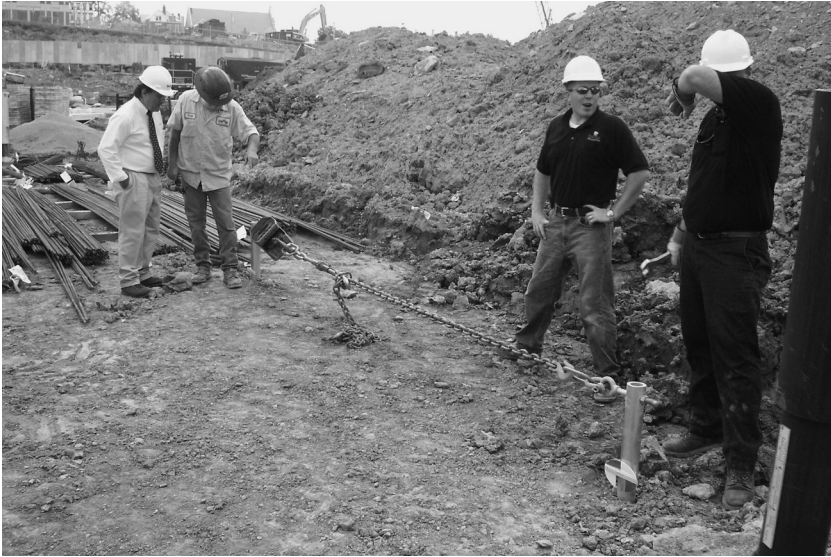
Figure 10.9 Lateral load testing on helical piles by pulling together (Courtesy of Magnum Piering, Inc.)
