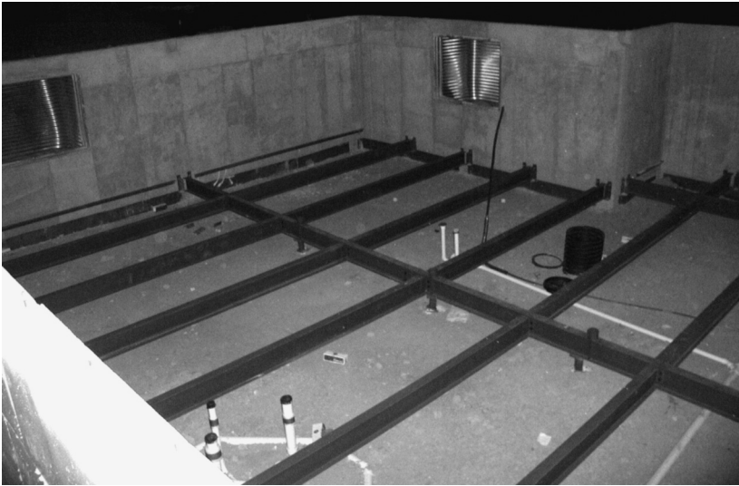
Figure 9.2 Structural floor construction on expansive soils
