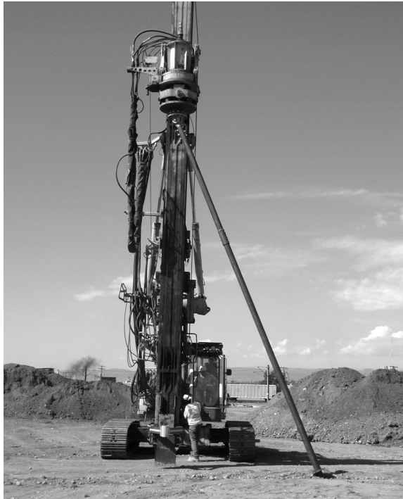
Figure 12.8 Installation of helical piles for parking garage (Courtesy of Hayward Baker, Inc.)
