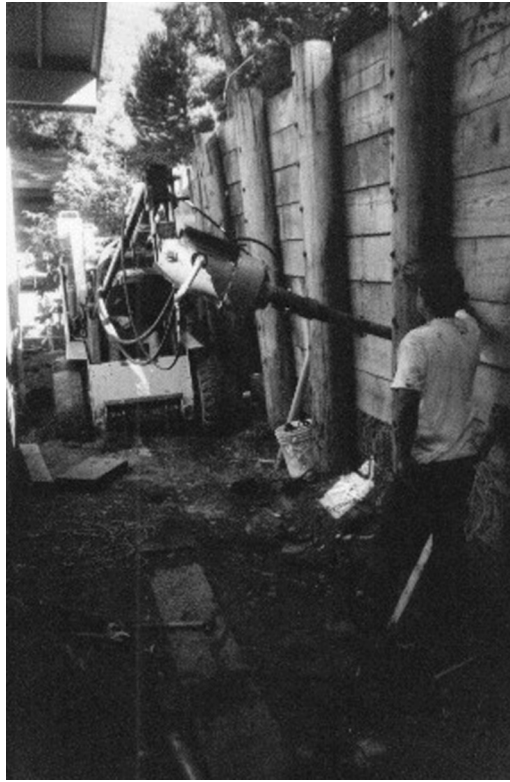
Figure 13.23 Repair of timber pile and lagging wall with helical anchors
