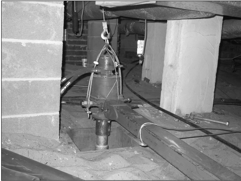
Figure 2.10 Low-headroom installation (Courtesy of Magnum Piering, Inc.)
