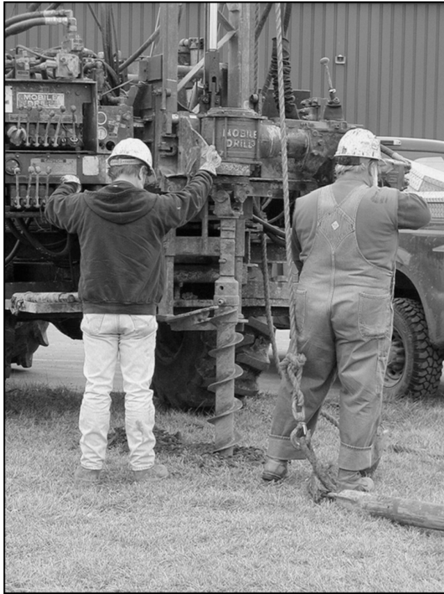
Figure 3.1 Typical soil boring rig with hollow stem augers
