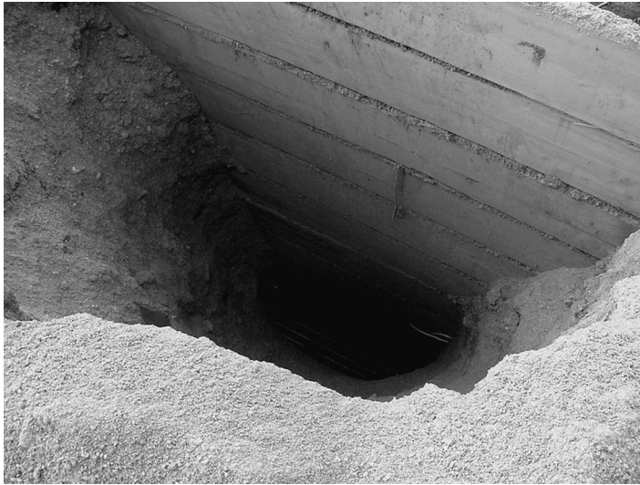
Figure 13.15 Soil silo formed by caving (Perko, 2008)
