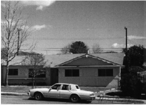
Figure 10.22 Residence, Northridge, CA (Rupiper, 2000)
