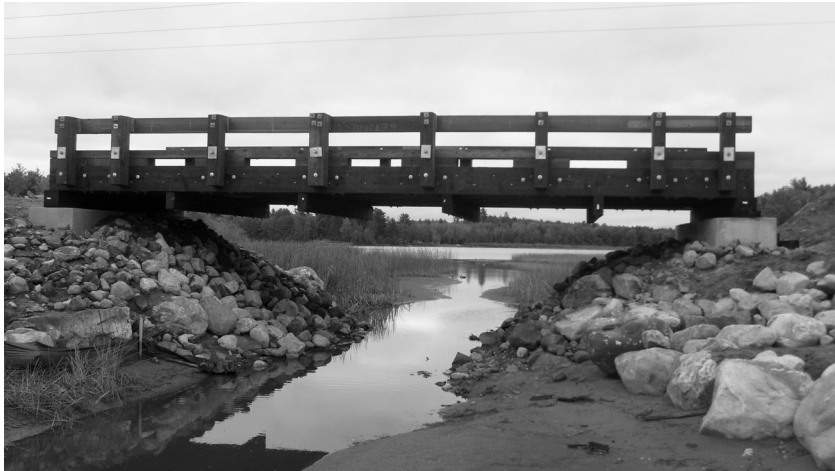
Figure 12.17 County bridge on helical foundation under construction
