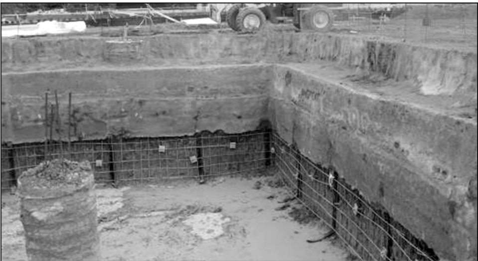
Figure 1.26 Shotcrete and helical anchor shoring system
