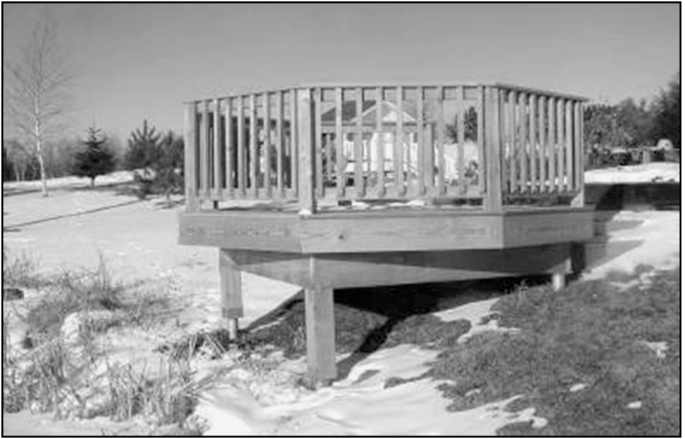
Figure 1.20 Deck and gazebo foundations (Courtesy of Magnum Piering, Inc.)
