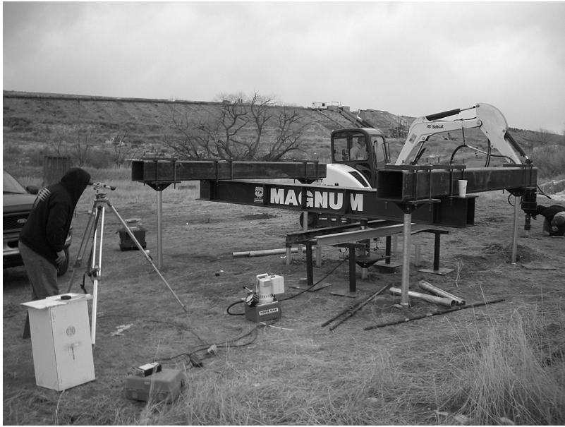
Figure 7.1 Example compression load frame (Courtesy of Magnum Piering, Inc.)
