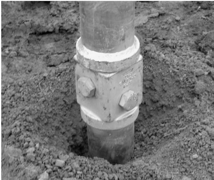
Figure 16.9 Square coupling (Courtesy of MacLean Dixie)
