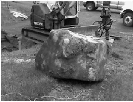
Figure 2.6 Removal of shallow obstruction (Courtesy of Magnum Piering, Inc.)
