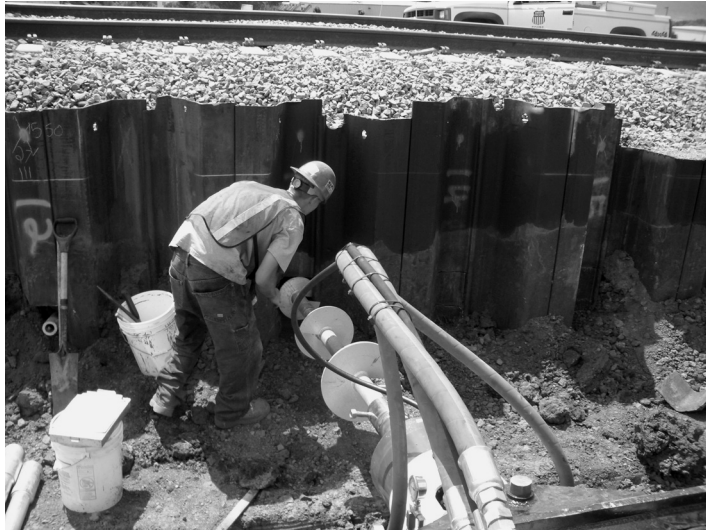
Figure 13.9 Installation of helical anchor for sheet pile wall (Courtesy of Magnum Piering)
