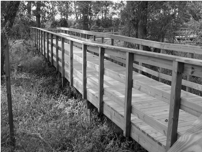
Figure 12.19 Boardwalk on helical piles
