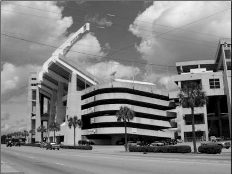
Figure 1.22 Stadium locker room addition
