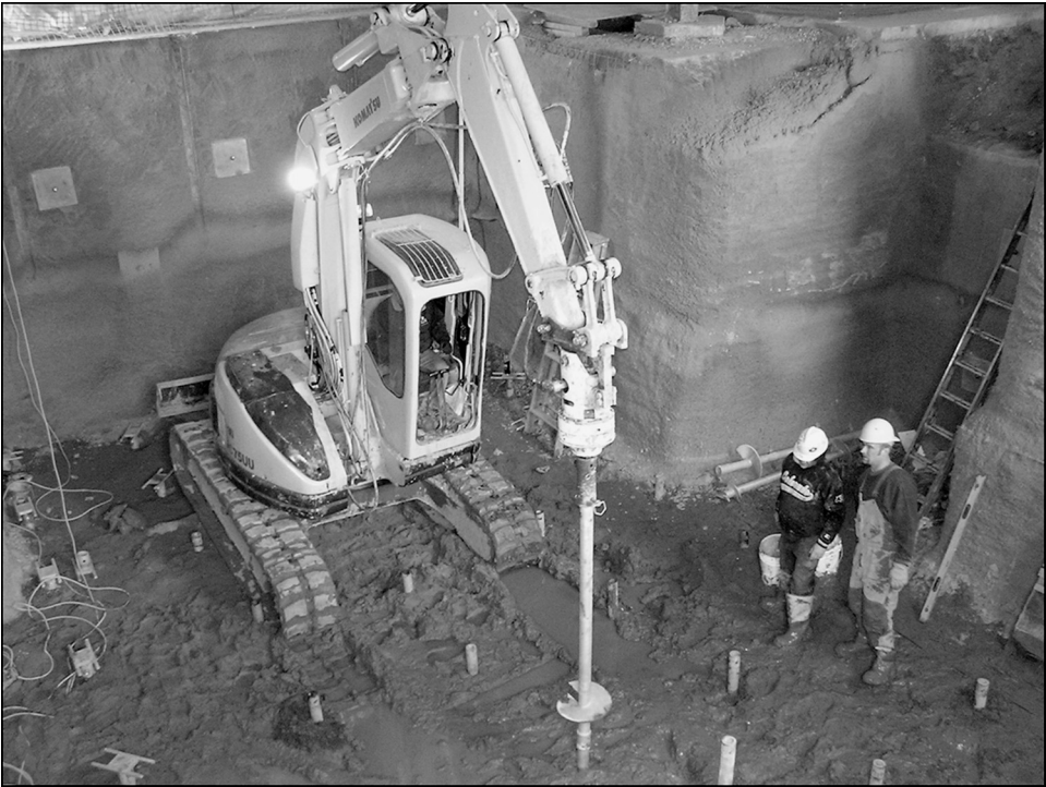
Figure 1.25 Helical pile foundation for underground MRI facility (Courtesy of Magnum Piering, Inc.)
