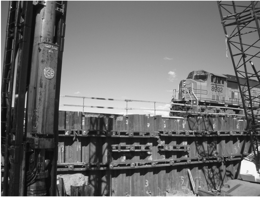
Figure 13.11 Union Pacific train passing over helical anchor wall (Courtesy of Magnum Piering)
