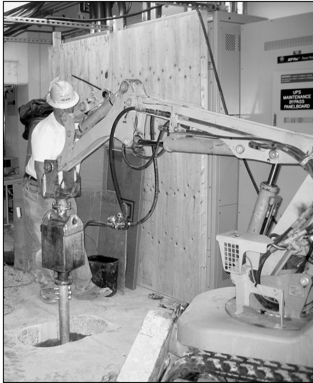
Figure 1.2 Helical pile installation in limited access area (Courtesy of Earth Contact Products, Inc.)
