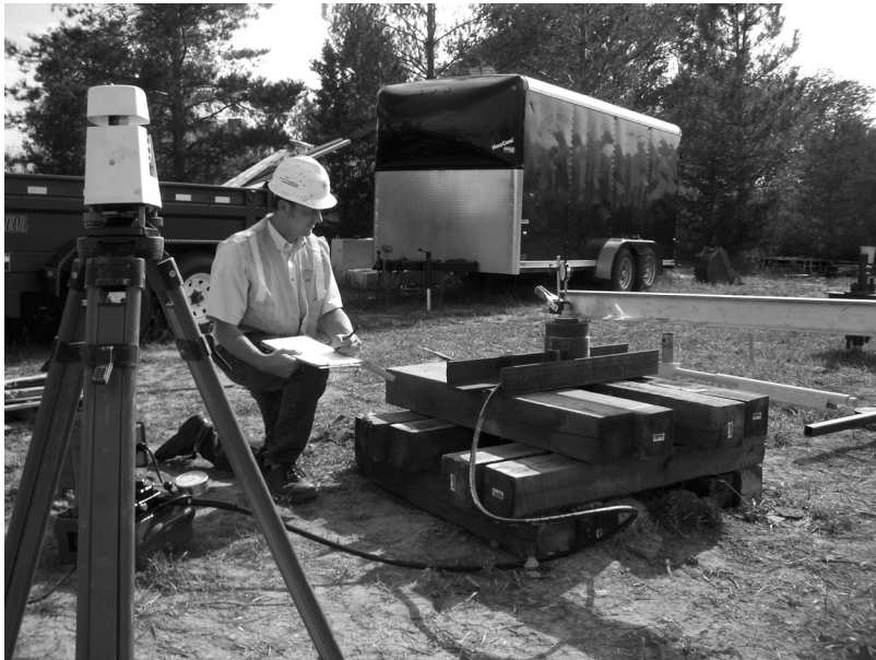
Figure 7.6 Helical pile tension test
