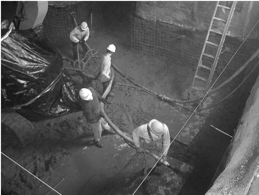
Figure 14.12 Shotcrete Application (Stage 3)
