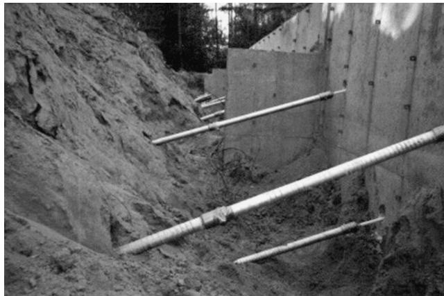
Figure 13.22 Repair of counterfort wall with helical anchors
