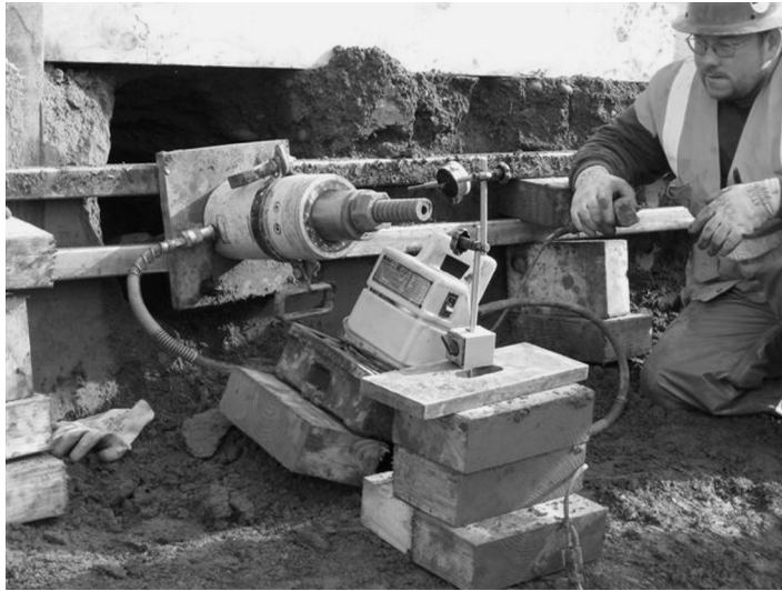
Figure 13.21 Helical anchor post-tension in progress (Courtesy of ECP)
