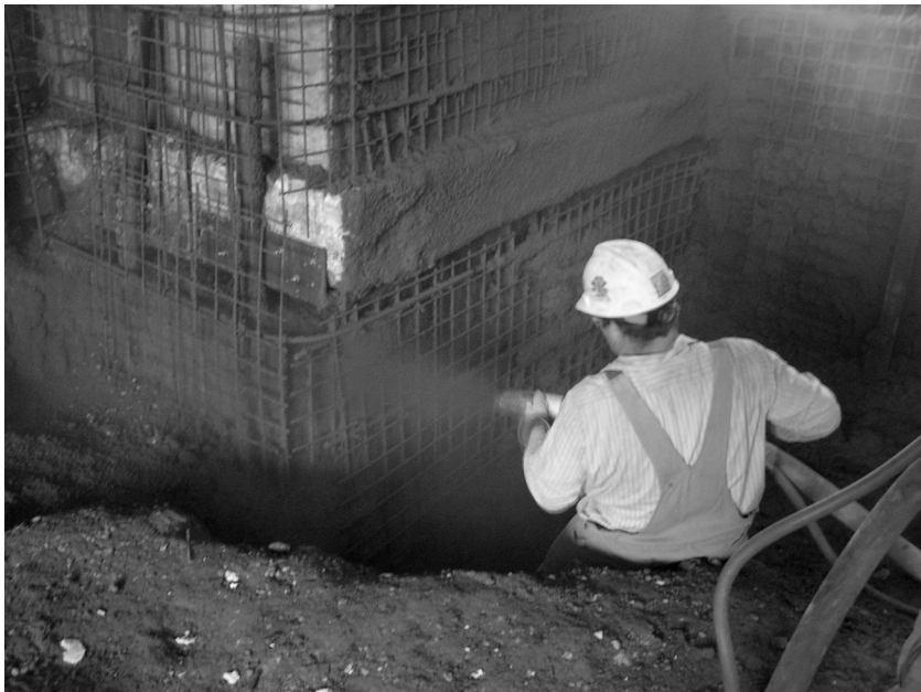
Figure 14.11 Shotcrete Application (Stage 2)
