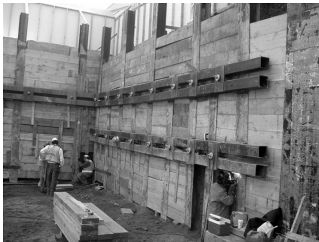
Figure 13.13 Soldier pile and lagging wall with helical tie-backs (Courtesy of ECP)
