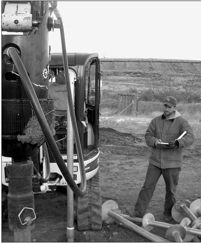
Figure 2.28 Helical pile inspection
