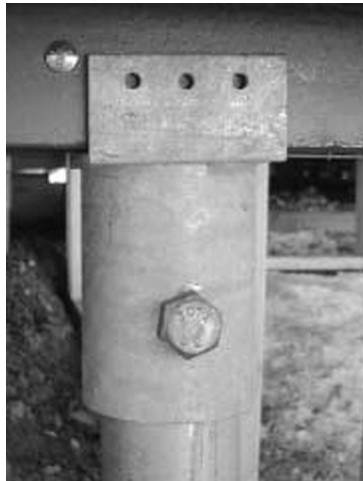
Figure 12.15 Example flitch beam cap
