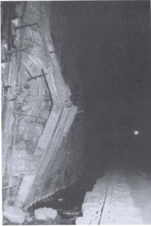
Figure 1.6 Heavily supported tunnel excavated by blasting.
