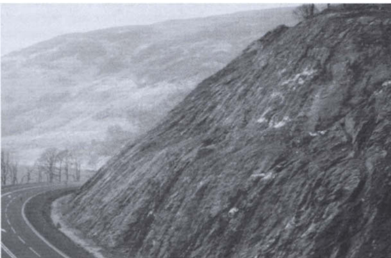
Figure 1.4 Example of a rock face made by pre-split blasting to give a stable, relatively smooth finish.
