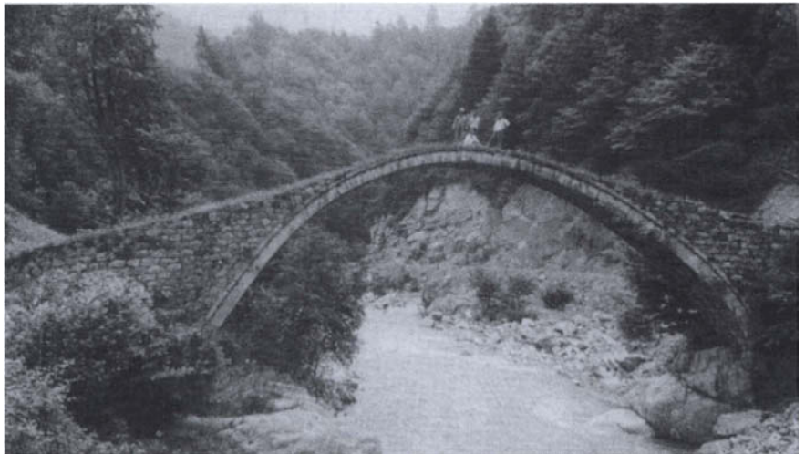
Figure 20.5 Masonry bridge demonstrating a voussoir arch comprised of a single set of rock blocks (northern Turkey).
