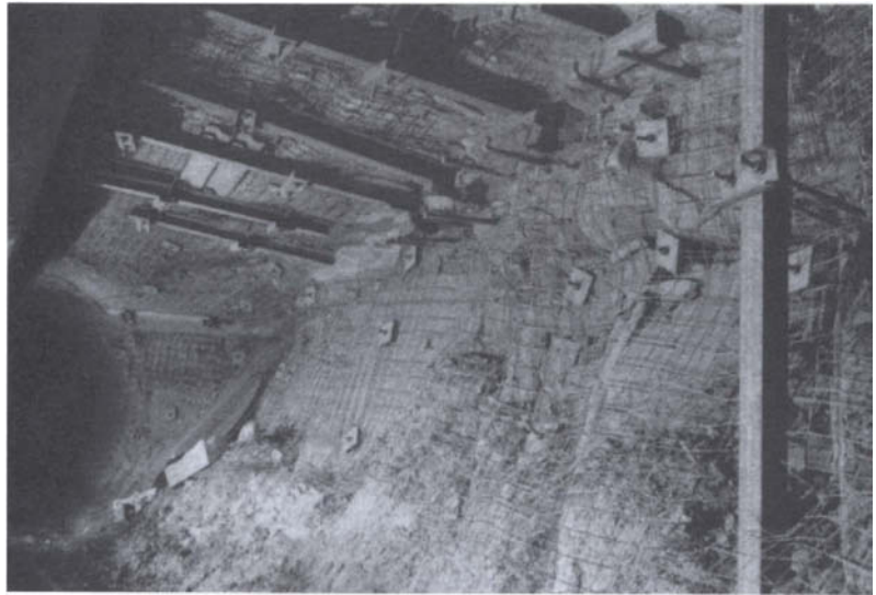
Figure 2.6 Tunnel in mudstone which has deteriorated over a period of several years after excavation.
