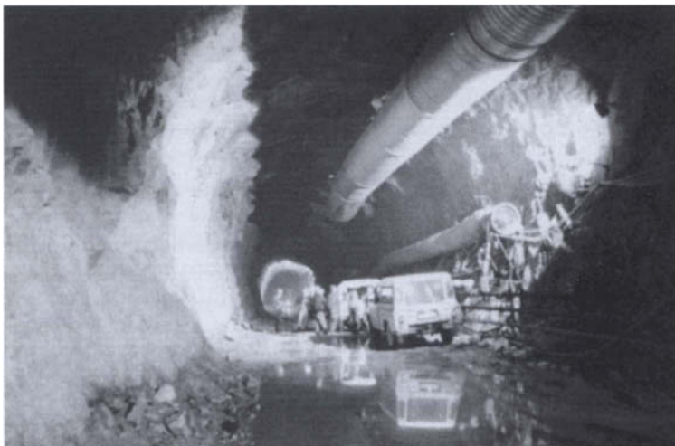
Figure 1.11 Hydroelectric cavern in Portugal.
