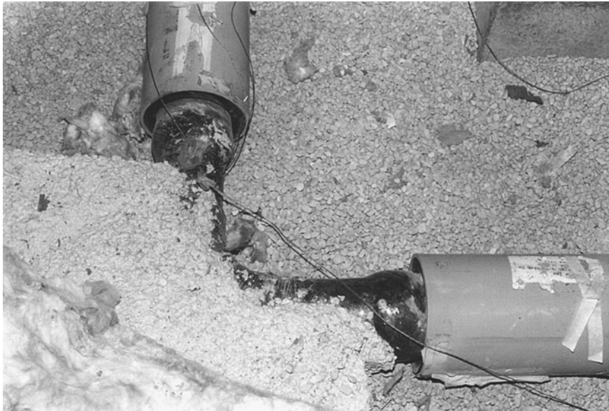
Figure 6.64 Elbow and thrust restraint for condensate pipe.
