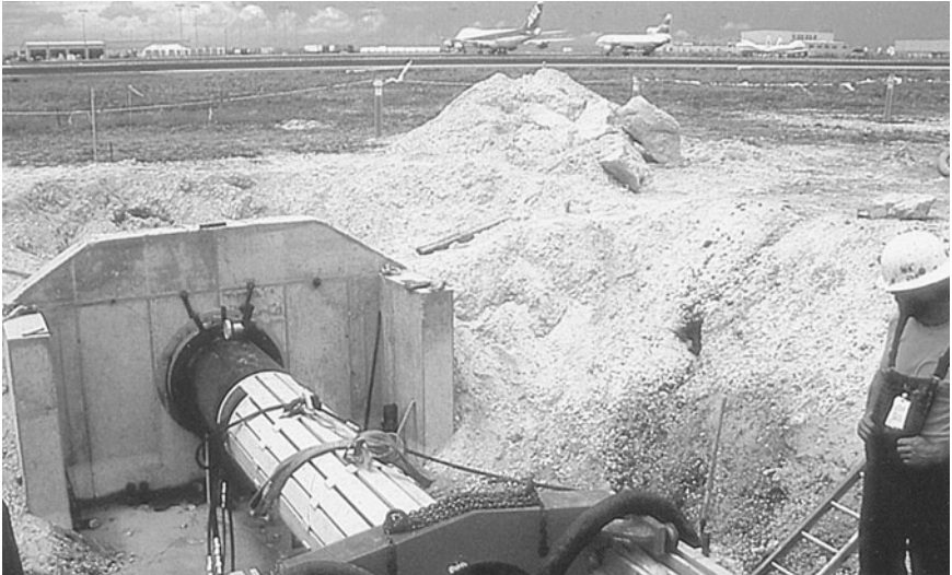
Figure 8.22 Completely unnoticed by the constant air traffic, microtunneling takes place directly under the active runway at the Honolulu International Airport. (Courtesy of Herrenknecht GmbH, Germany.)
