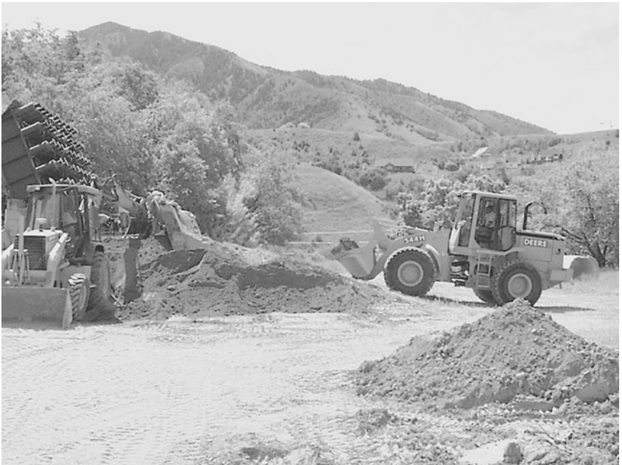
Figure 7.59 Soil placement process.
