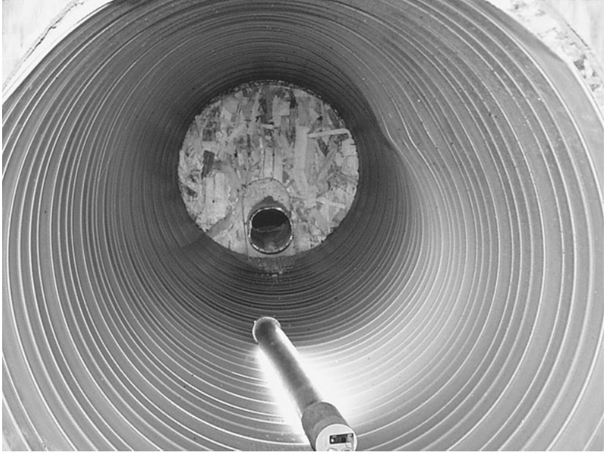
Figure 6.23 Small inversion in sidewall due to 16,000-lb live load adjacent to pipe. Pipe installed with 1 ft of cover.
