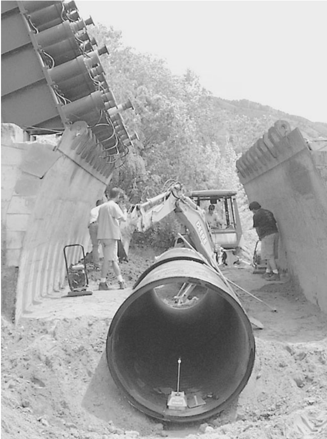
Figure 7.57 Soil placement, compaction, and density measurement.
