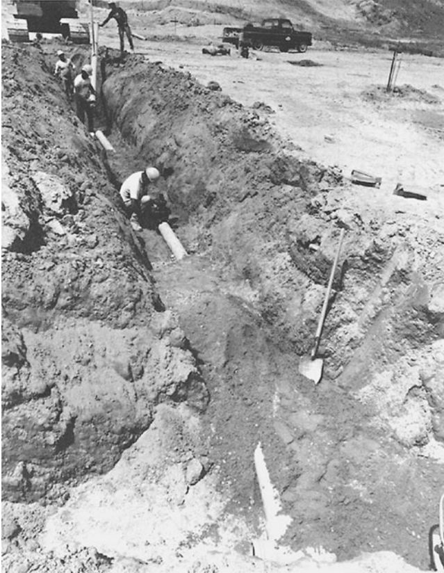
Figure 7.1 PVC's high strength-to-weight ratio is a real advantage. (Reprinted by courtesy of Uni-Bell PVC Pipe Association.)
