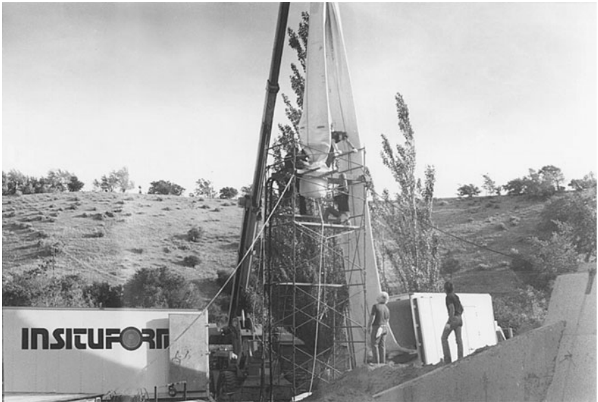
Figure 8.4 Equipment for inverting the Insitutube.
