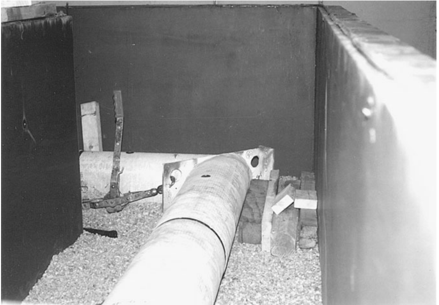
Figure 6.61 Elbow with steel anchor plate before concrete thrust block was cast in corner.
