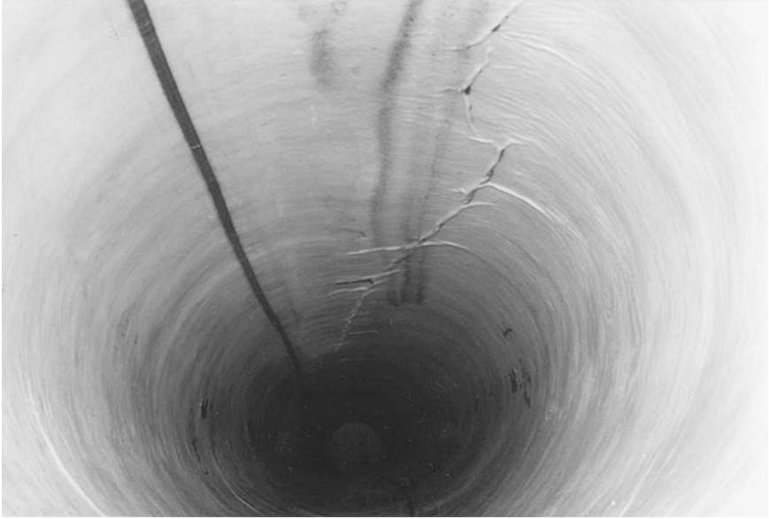
Figure 8.9 The inside of the lined broken rigid pipe test section. The vertical soil pressure is 8700 \text{ lb/ft}^2 .
