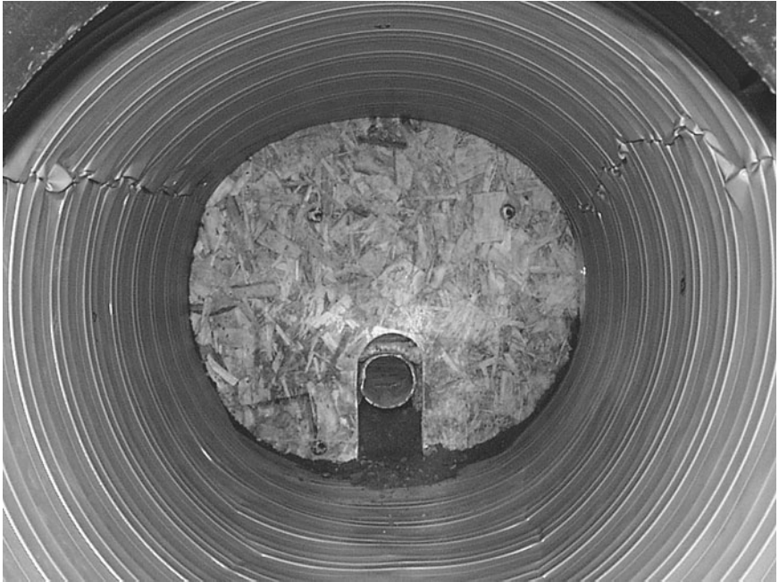
Figure 6.41 Steel-ribbed pipe (30-in diameter) at 60 ft of cover in silty-sand soil at 97 percent density.
