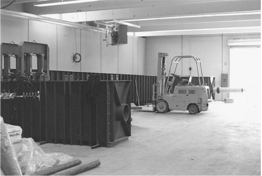
Figure 6.55 Test facility under construction. Foreground: soil load cell; center to rear: water infiltration test cell.
