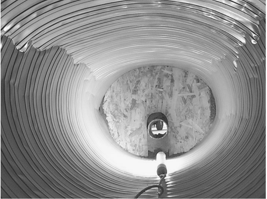
Figure 6.39 Steel-ribbed pipe (24-in diameter) at 49 ft of cover in silty-sand soil at 91 percent density.
