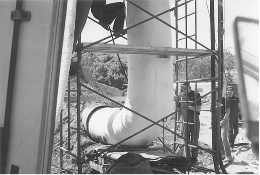
Figure 8.5 Process of inverting the Insitutube.
