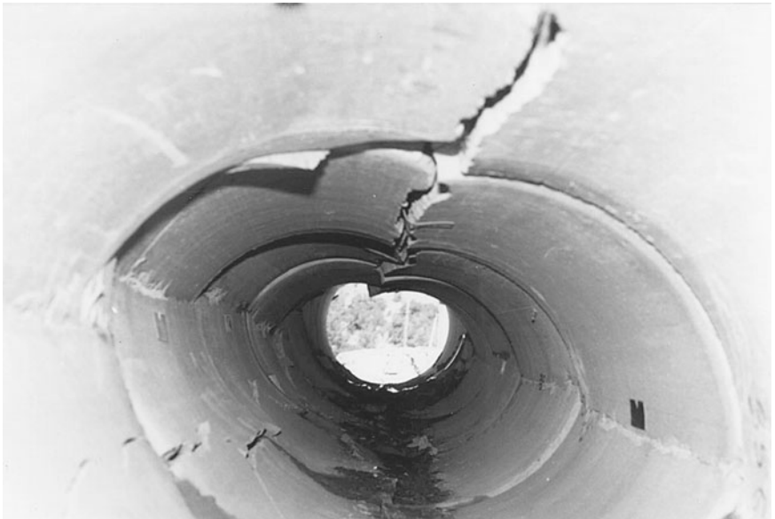
Figure 8.8 The inside of the lined broken rigid pipe test section. The vertical soil pressure is 5040 lb/ft 2 (equivalent burial depth of 42 ft).
