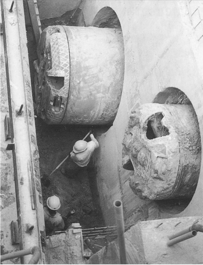
Figure 8.23 Parallel-drive microtunneling machines are right on target as they enter the receiving pit in Dubai. (Courtesy of Herrenknecht GmbH, Germany.)
