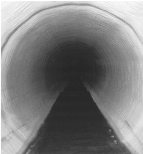
Figure 8.14 Portrayal of the folded pipe as inserted and how it appears after expansion. (Courtesy of Ultraliner.)
