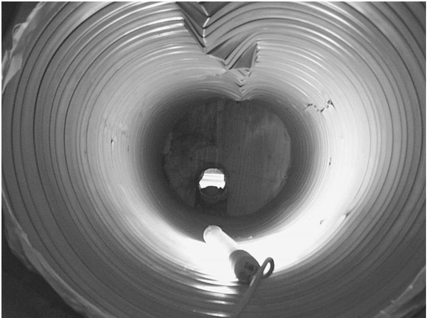
Figure 6.33 Steel-ribbed pipe (18-in diameter) at 75 ft of cover in silty-sand soil at 95 percent density.
