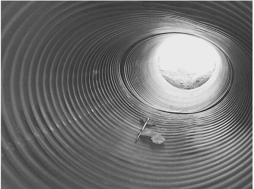
Figure 7.69 Local buckling at 5 o'clock. Density = 77 percent, and load is 46 ft of cover.
