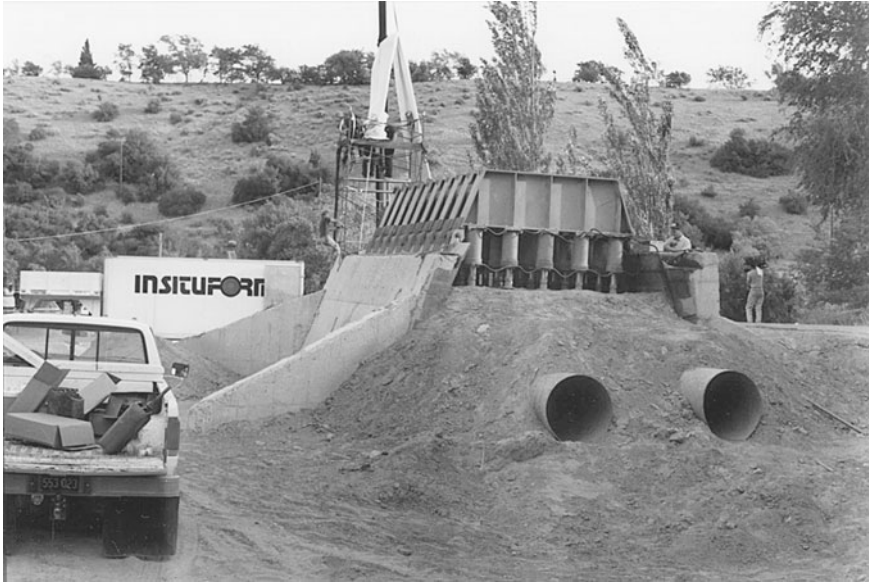
Figure 8.2 Test sections of pipe in place showing the process of inserting the Insituform pipe. The pipes visible are access pipes.
