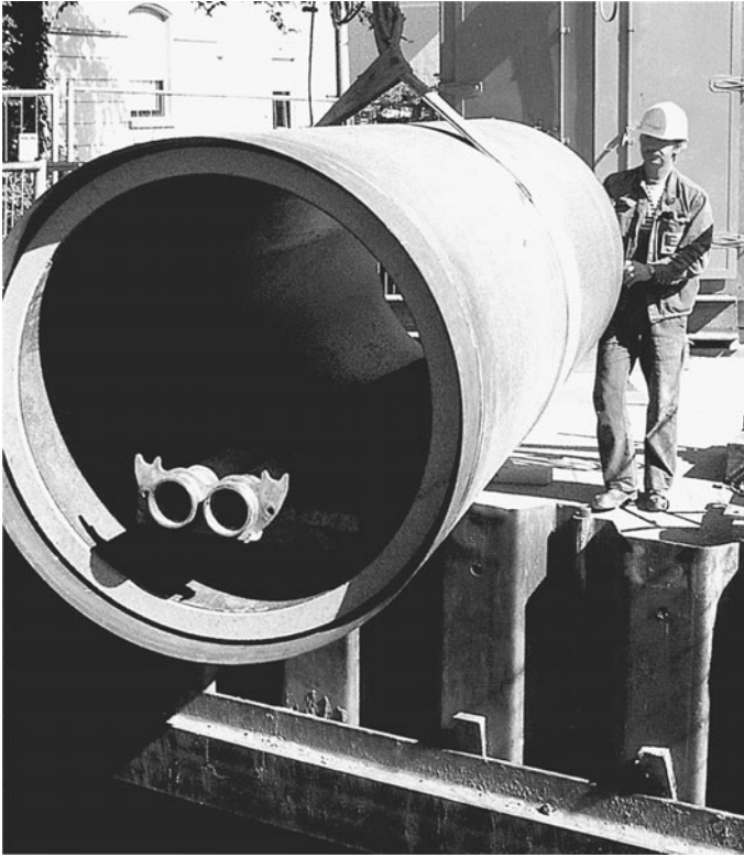
Figure 8.17 Polycrystalline pipe is being placed in the jacking pit. Note prepackaged tubes for supplying fluid to boring machine and removing slurry. (Courtesy of Meyer-Polycrystalline.)
