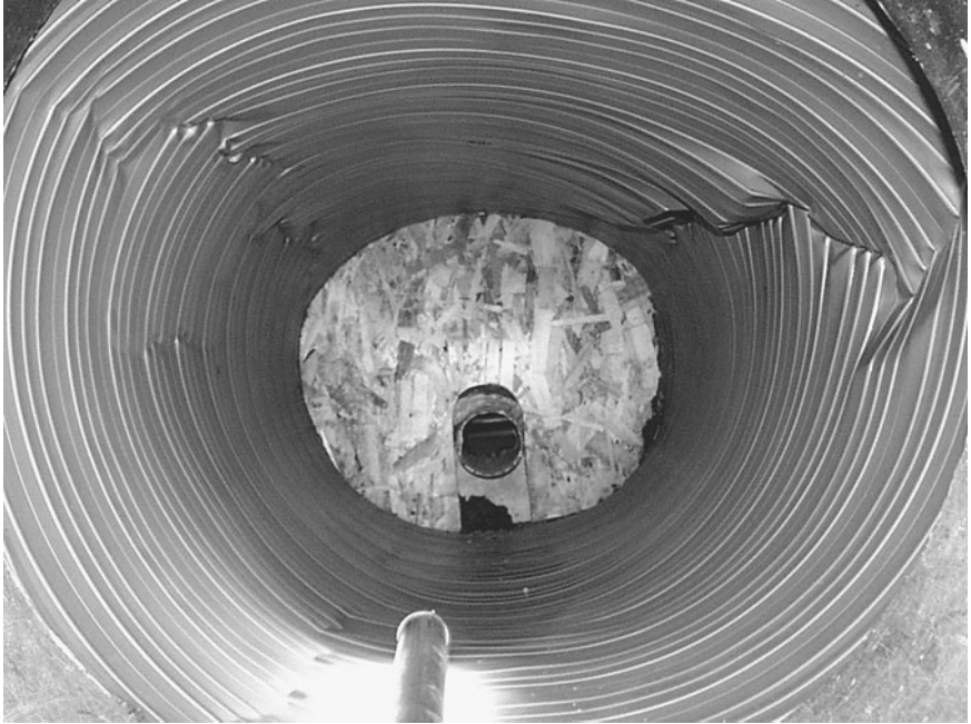
Figure 6.37 Steel-ribbed pipe (24-in diameter) at 43 ft of cover in silty-sand soil at 95 percent density.
