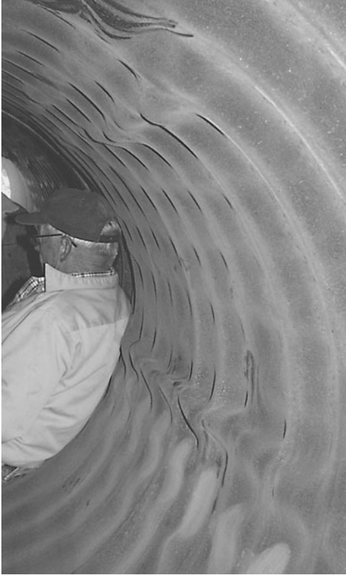
Figure 7.75 Wall crushing and dimpling pattern on right side. Density = 95 percent and load is 152 ft of cover.
