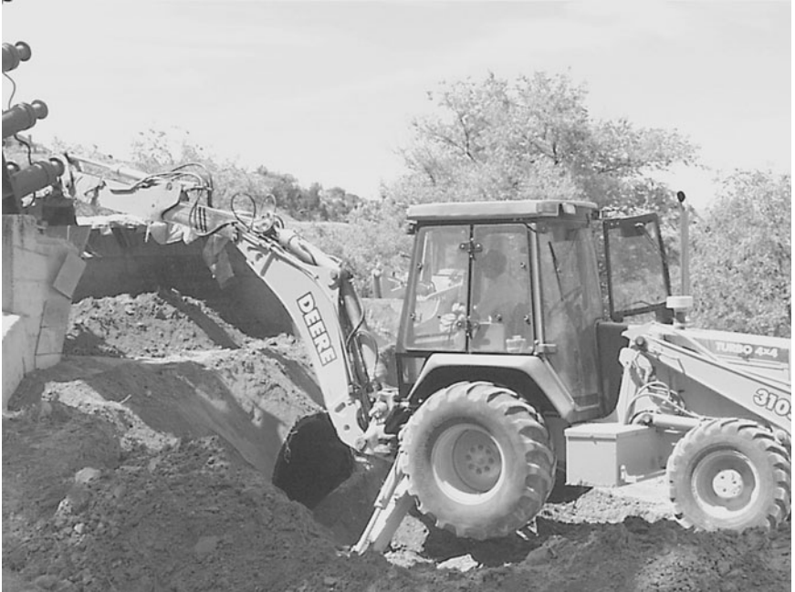
Figure 7.58 Backhoe loading soil in test cell.
