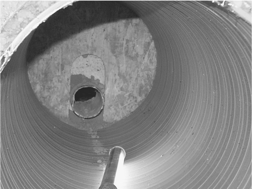
Figure 6.32 A 24-in pipe, with 2 ft of cover, showing no adverse reaction to a 16,000-lb live load.
