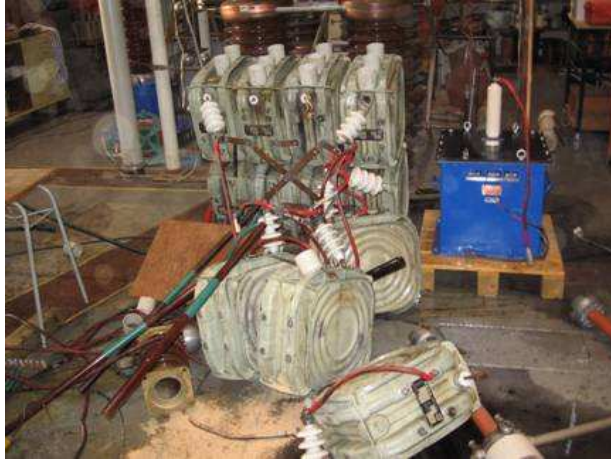
(a) Multiple capacitor failure due to electrical fault of a single capacitor.
