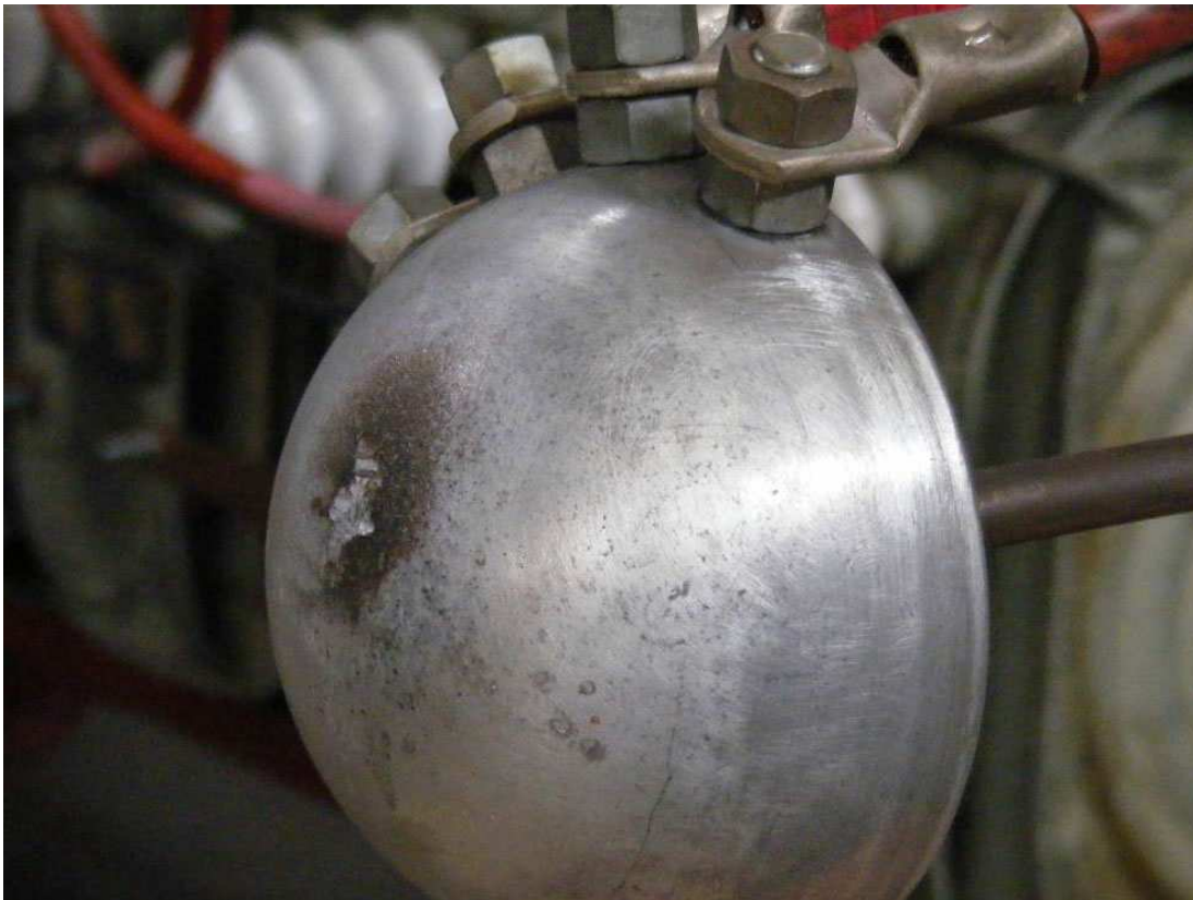
Figure 5.20 Pitting from high current arcing on the 125mm spheres used on the switch
