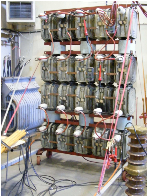
(a) Completed capacitor bank with strops and wiring
