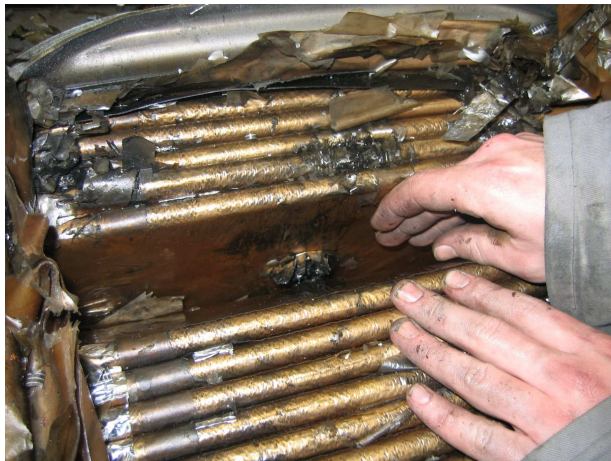
(c) Internal foil layers showing the area under fault.
