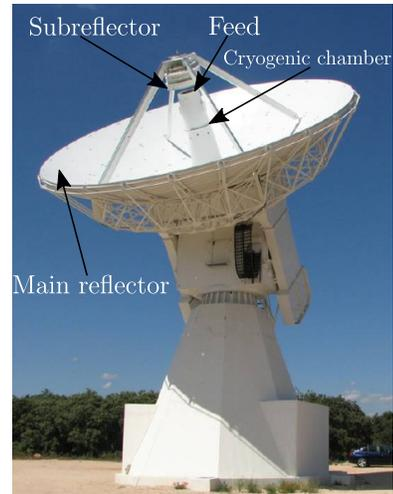
Fig. 1. The VGOS 13m radio telescope in Yebes, Spain.
