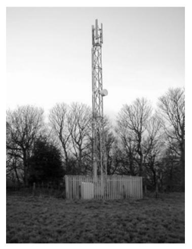
Figure 6.12 Tower-mounted sectored antennas (Courtesy of BT)
