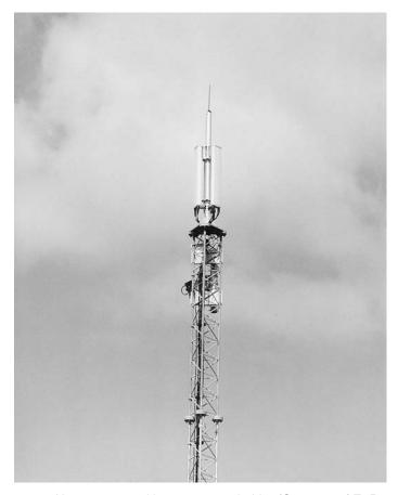
Figure 6.23 Narrow tower without separate ladder (Courtesy of E. Randall)
