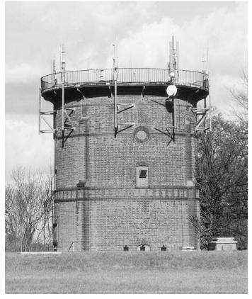
Figure 6.21 Roof mounted equipment - round brick tower (Courtesy of E. Randall)
