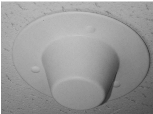
Figure 24.21 Typical ceiling-mounted indoor antenna.
