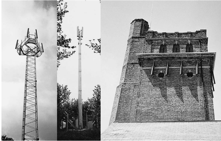
Figure 24.17 Typical macrocell installations.
