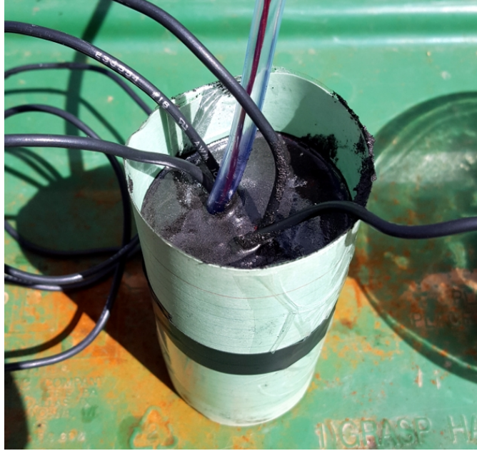
Figure 14g: Casting the 1:1 transformer. Plastic-tape-coated cardboard is used here to allow for some over-fill.
