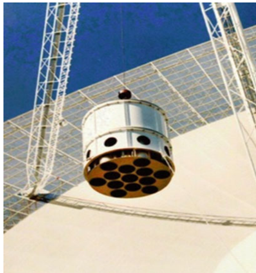
Fig. 19 L-band multibeam feed lifted into position on Parkes radio telescope (Picture: courtesy of CSIRO Australia)
