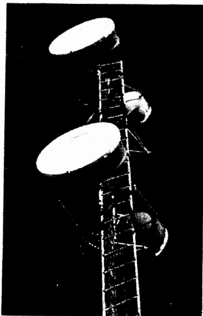
FIG. 30-1 Typical tower with radio relay antennas. (Courtesy Andrew Corp.)
