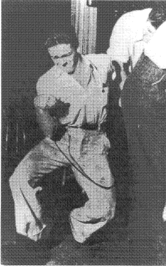
FIGURE 8.8. An experiment subject undergoes let-go current threshold testing. (From Dalziel, (©) 1972, IEEE.)
